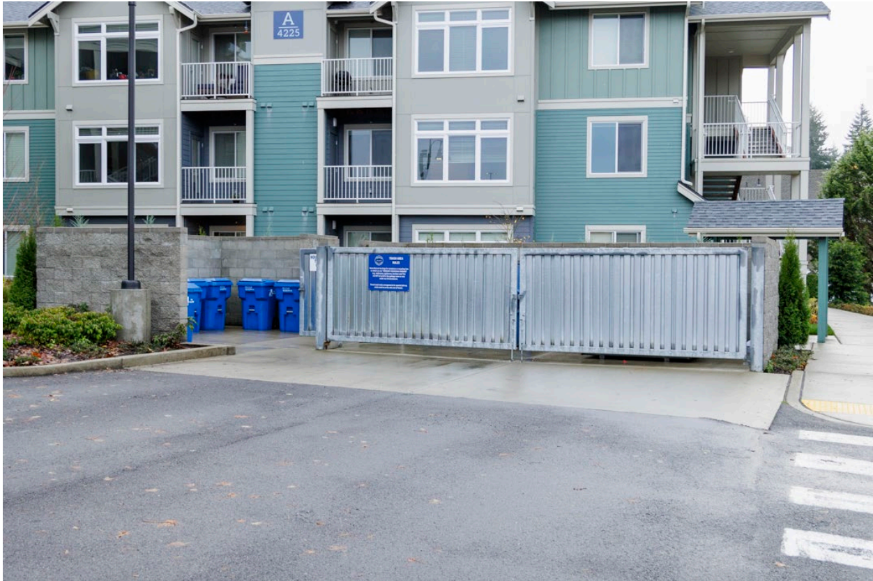
Figure 6 Multi-Family Collection Site
