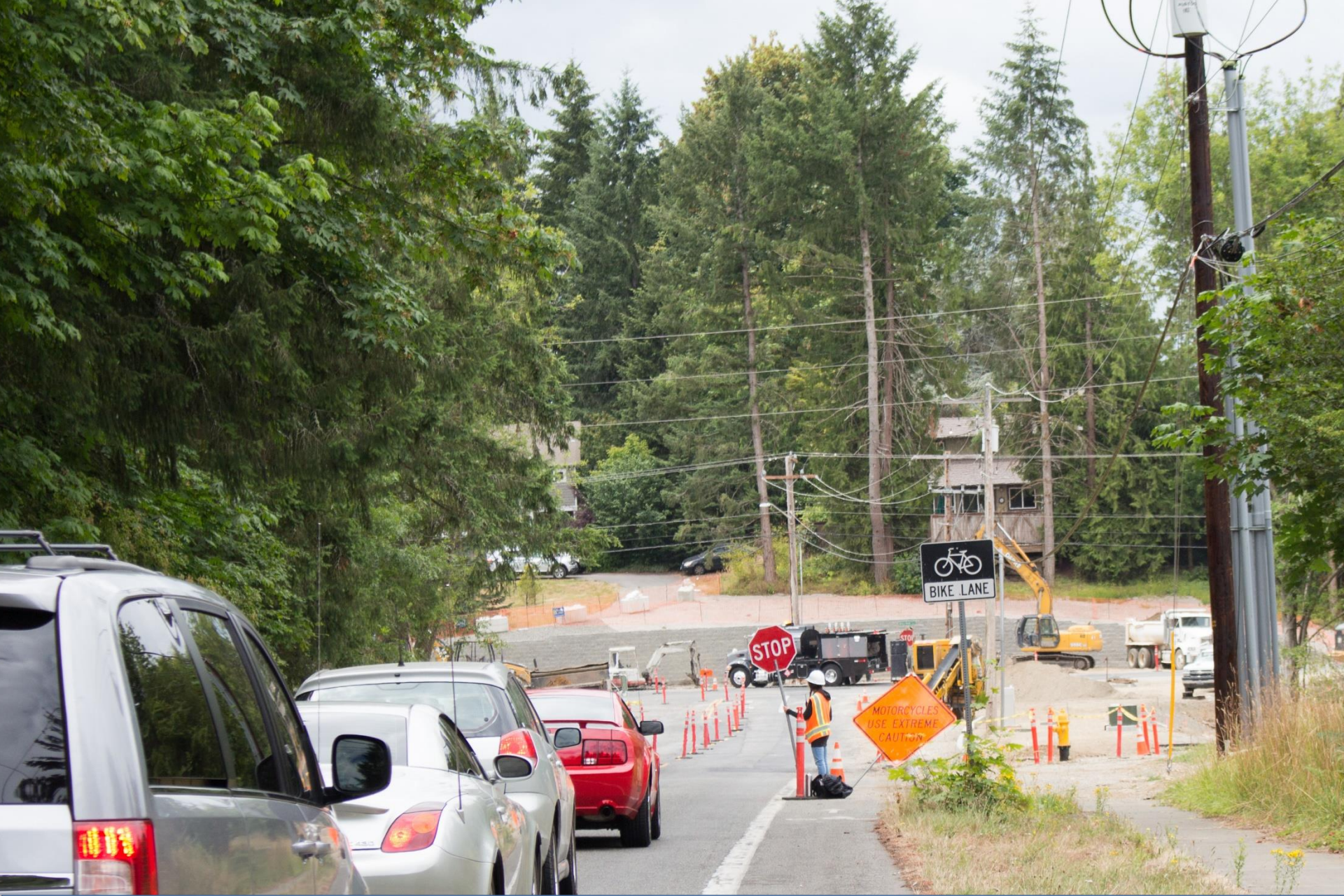
Boulevard Morse-Merryman Roundabout
