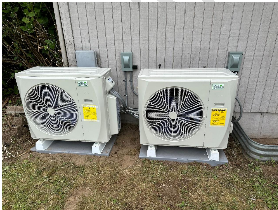
Heat pump outdoor units are installed at a home in Olympia.
