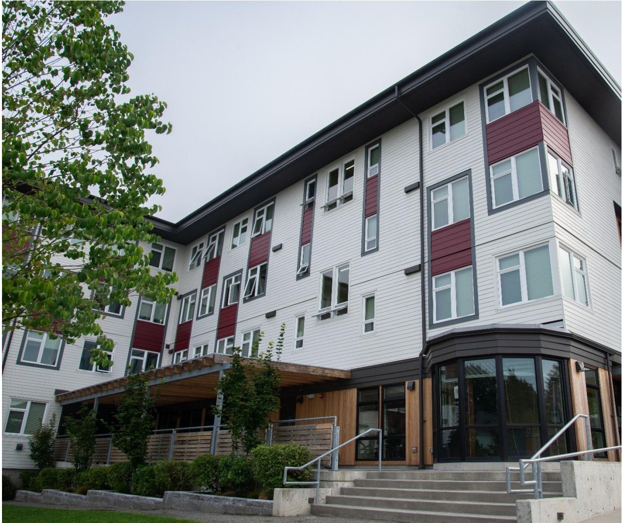
An apartment complex providing emergency and permanent supportive housing in Olympia.
