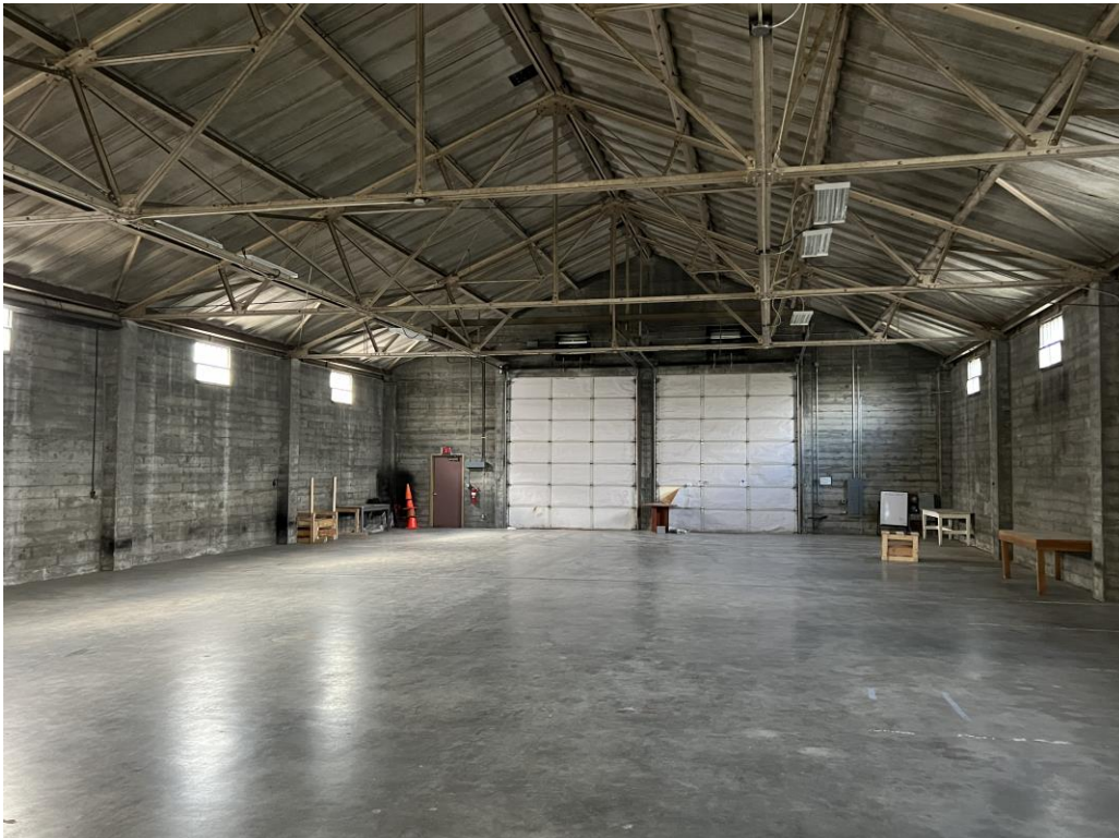
19 of 22 (WA_Thurston_NationalGuardArmoryOlympia_0011) Interior view of the Vehicle Storage Building looking south.
