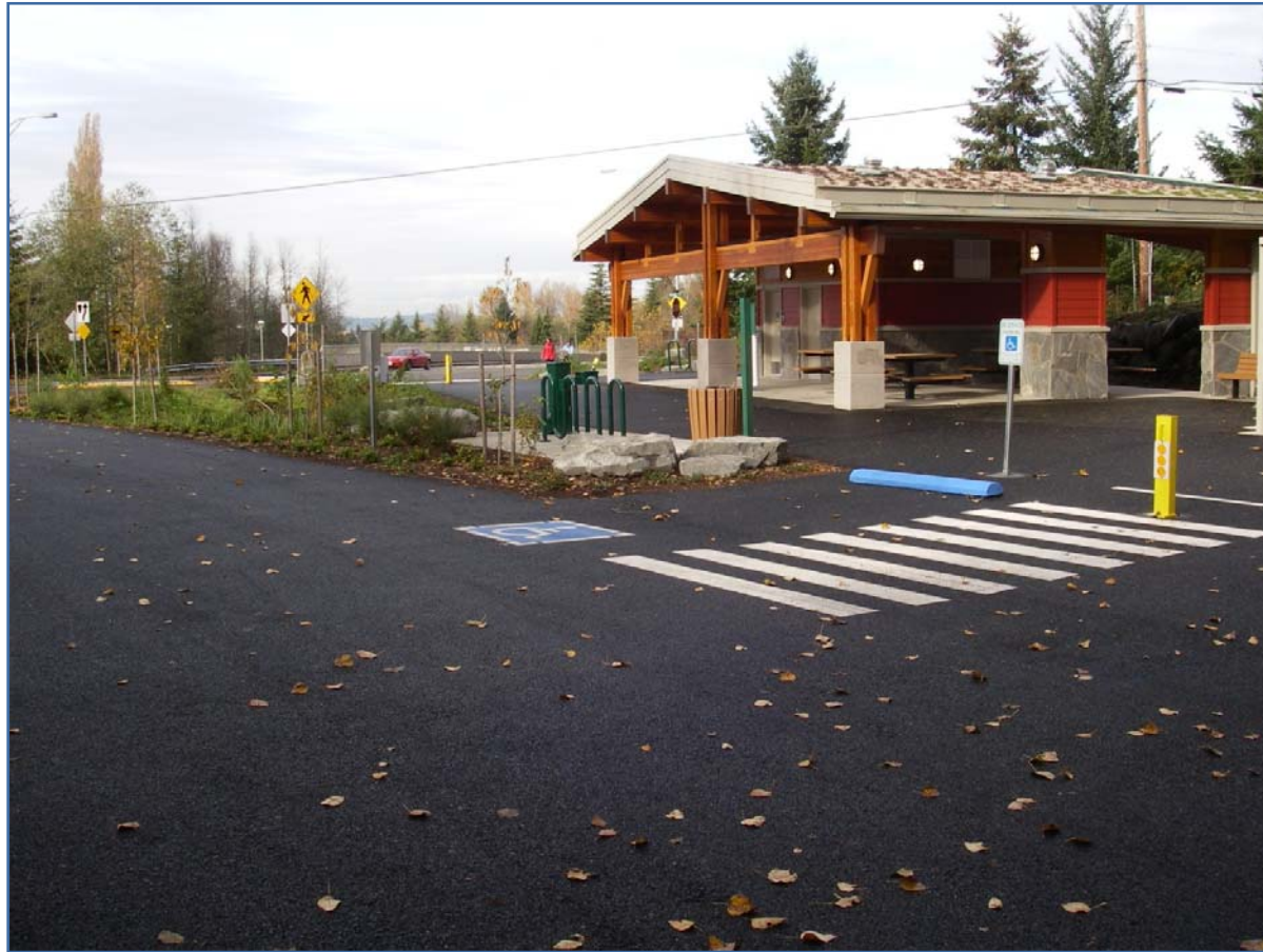
Olympia Woodland Trailhead: Features a living roof, a rain garden, and porous pavement.
