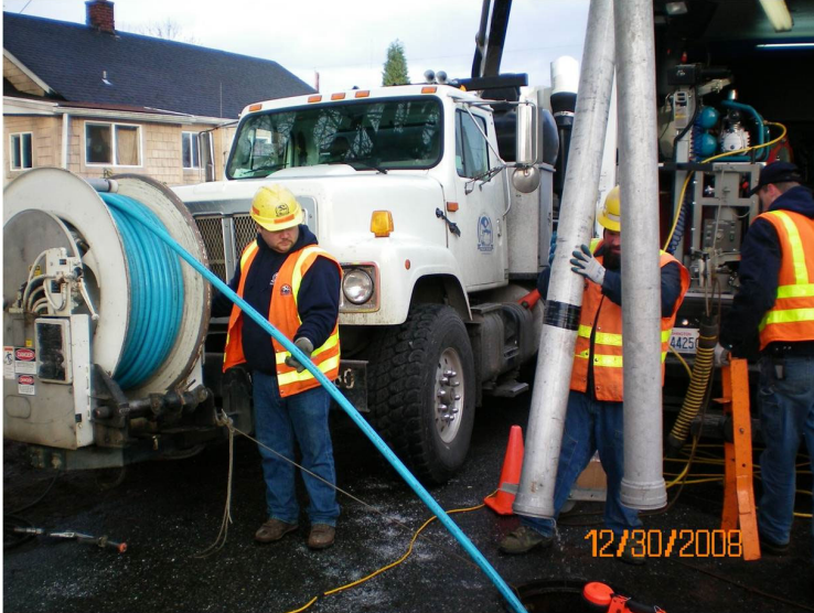
Olympia crew members maintaining the sewer system to ensure proper functioning.
