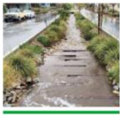
C Green stormwater infrastructure
