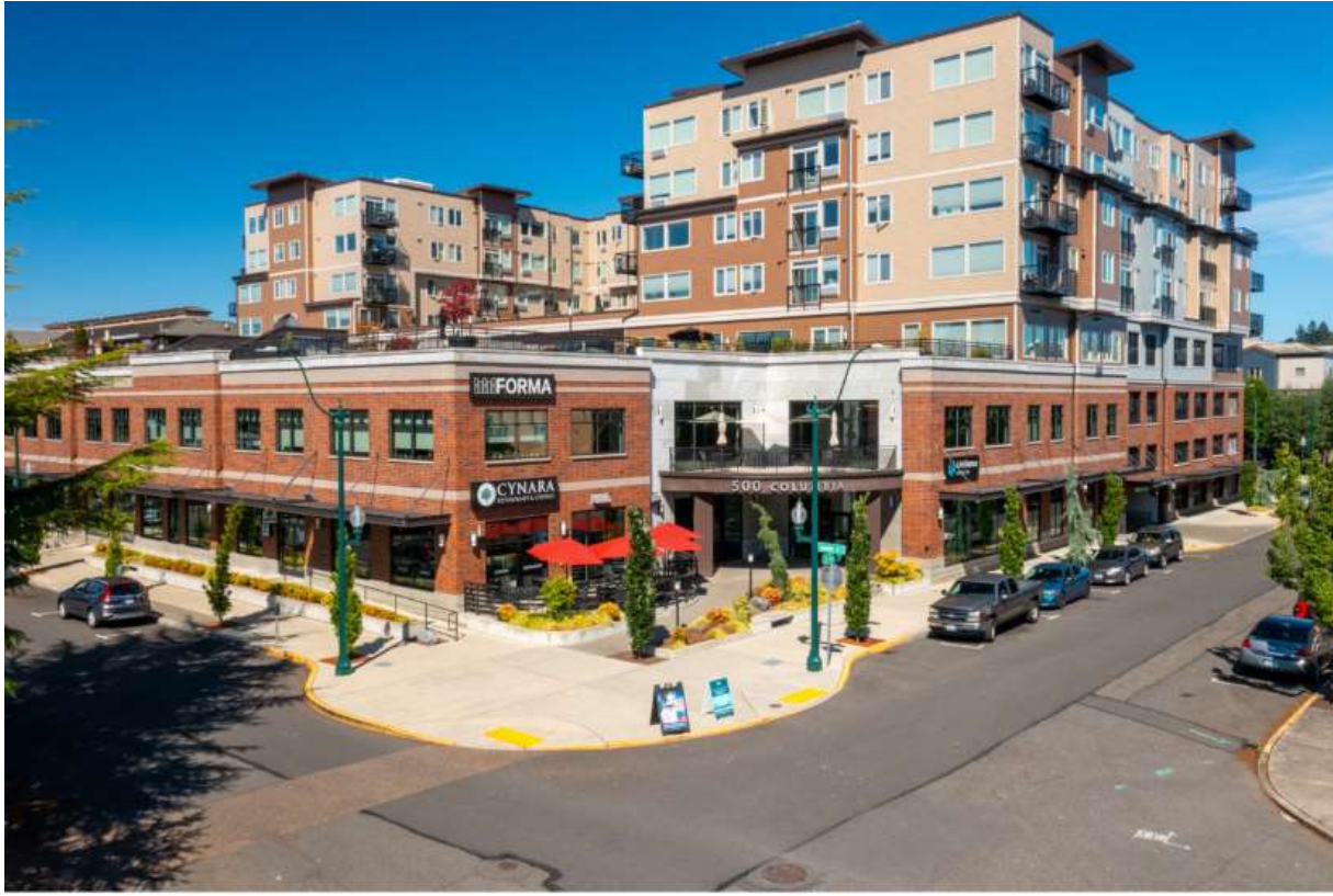
Bulb-out and streetscape built with new development in north downtown.
