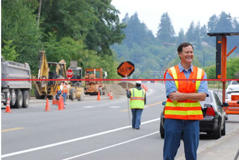
RW Johnson Boulevard is rebuilt.
