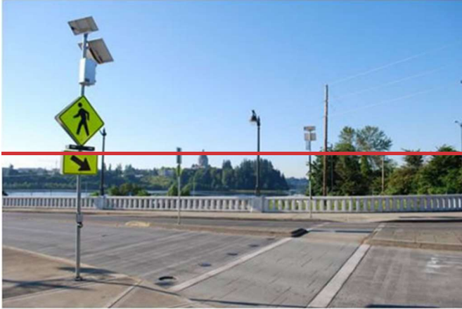
A flashing beacon at a crosswalk on Olympic Way will alert motorists to pedestrians.
