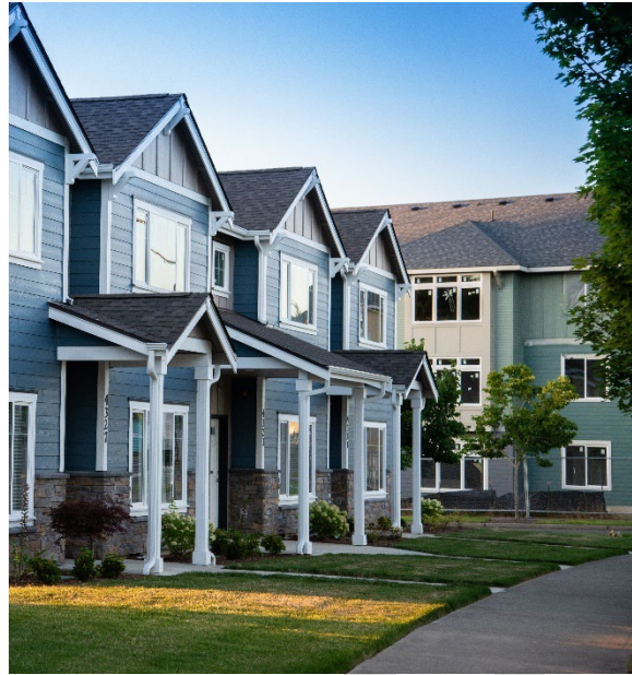
An Olympia neighborhood with a mix of apartments and town homes.
