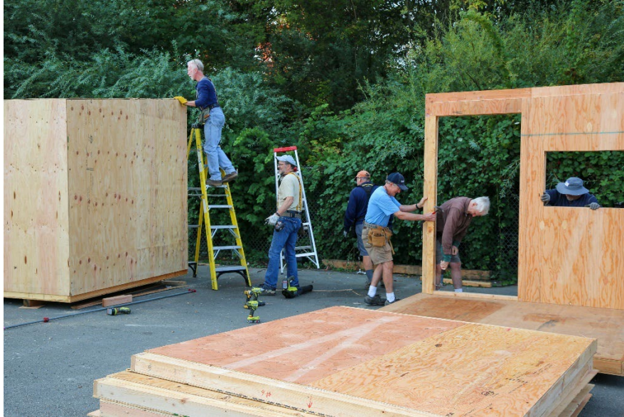
Community volunteers help build tiny homes for Quince Street Village.
