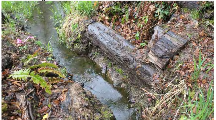
Photo 66. Cut channel and armored bank
