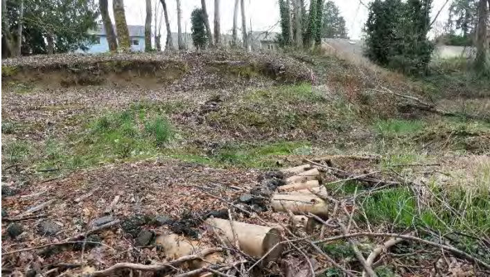
Photo 43. Cut slopes and wetland fill
