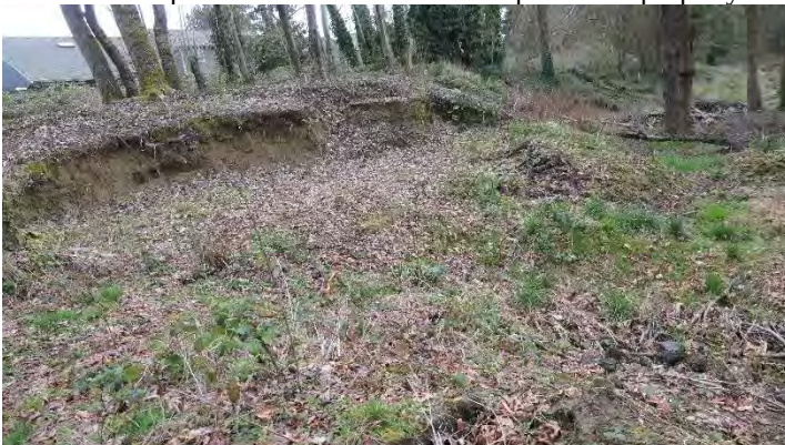
Photo 47. Cut slopes in wetland buffer
