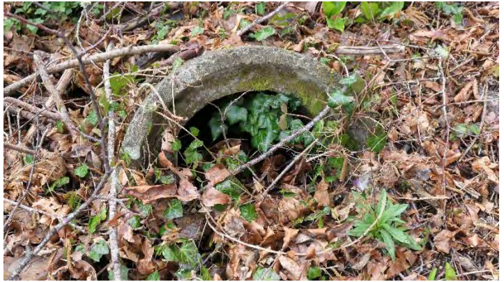
Photo 42. Concrete trash in Wetland A and buffer
