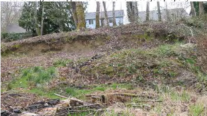
Photo 7. Cut material from slopes pushed into wetland
