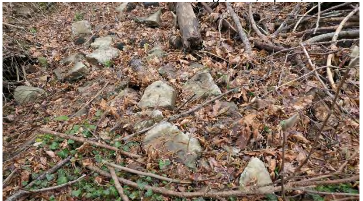
Photo 38. Concrete chunks in Wetland A
