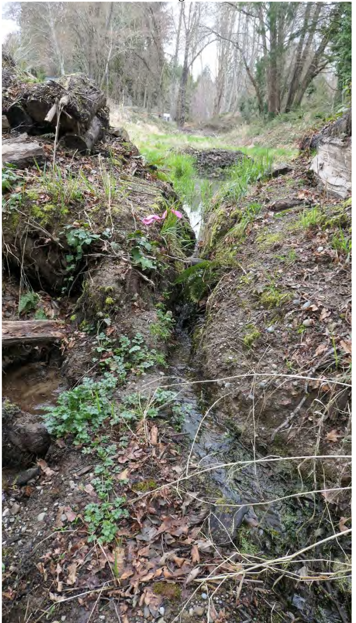
Photo 60. Excavated ditch draining Wetland A
