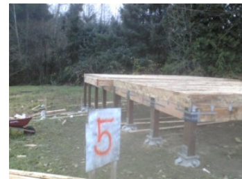
LID Foundation at Clearwater Commons in Bothell.
