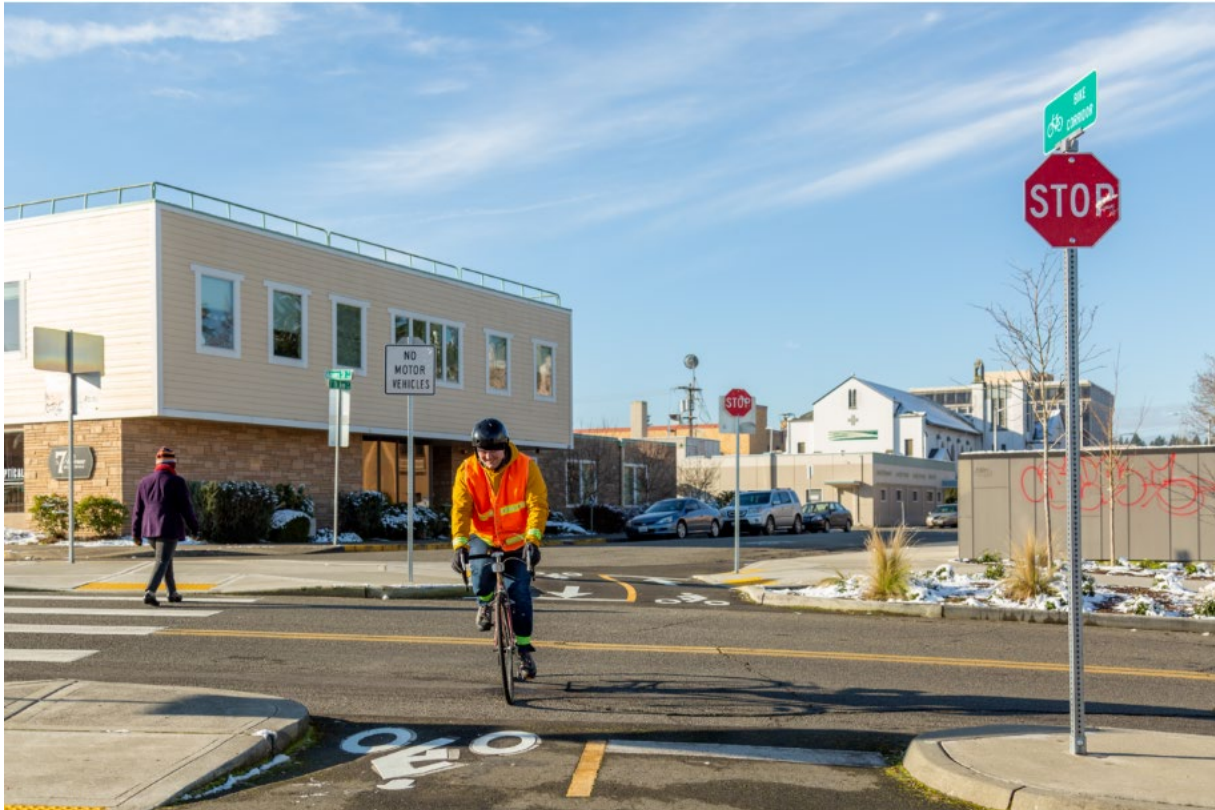
A bicycle-only crossing on 7th Avenue at Jefferson Street, which also includes a marked crosswalk for pedestrians with ADA compliant curb ramps.
