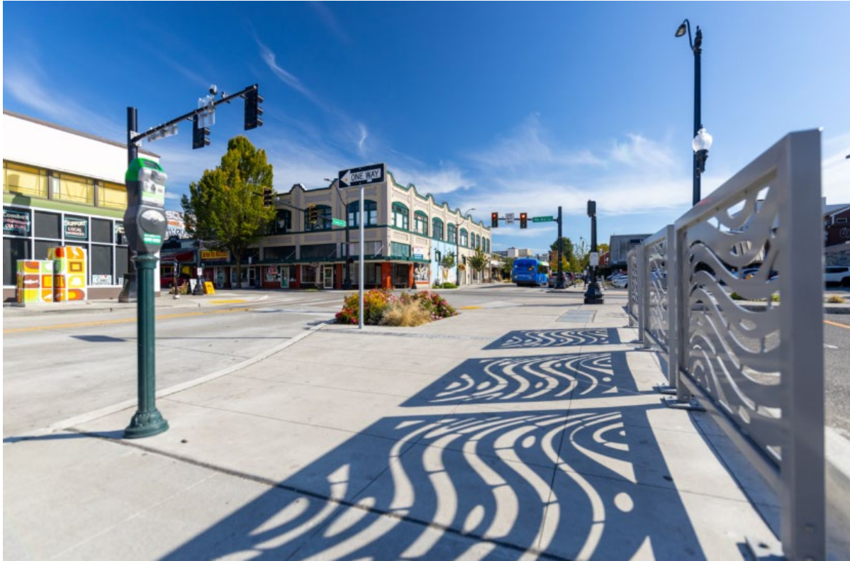
The rebuilt sidewalk on Franklin Street included some public art elements to make walking more inviting.
