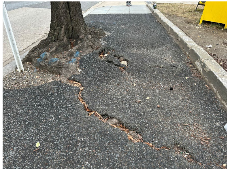
Rubberized asphalt installed in Washington DC about 10 years post-installation
