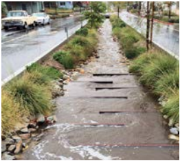
C Green stormwater infrastructure
