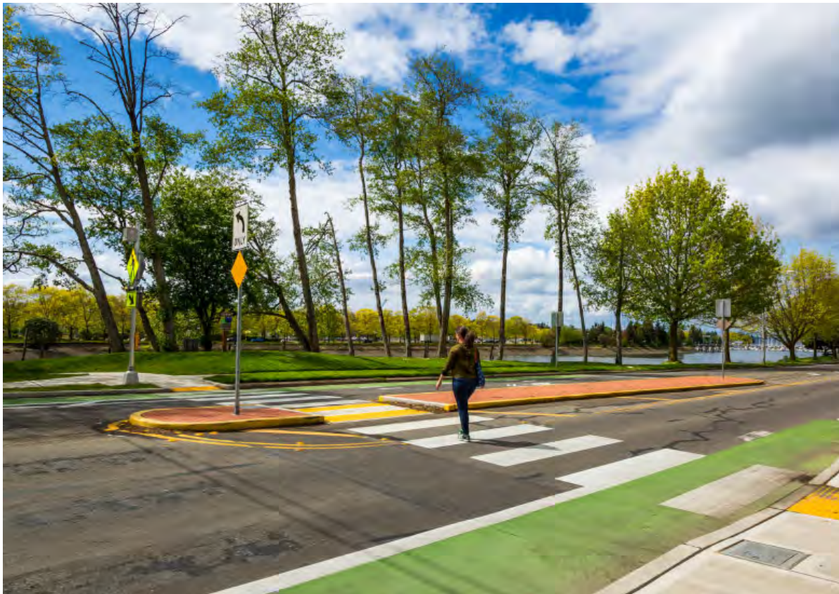
The flashing beacons, island, and crosswalk marking make crossing East Bay Drive at Olympia Avenue safer and more inviting.
