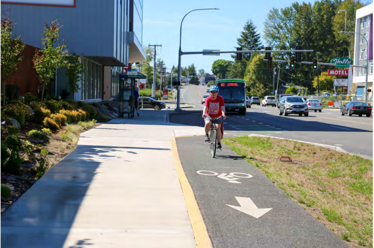
A bicyclist rides down the 4th Avenue Bridge in the separated bike lane on Martin Way, which is one kind of enhanced bike lane.
