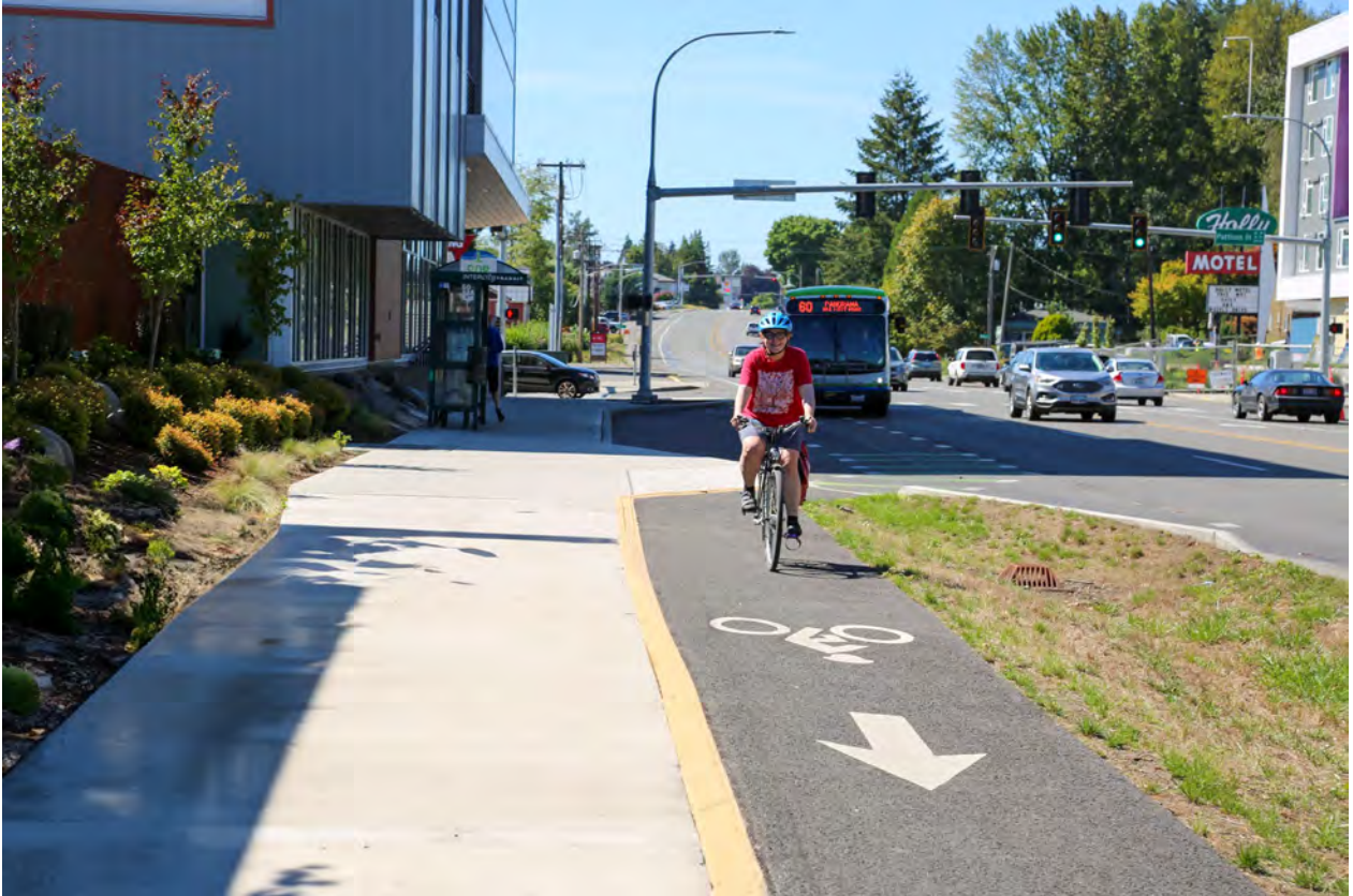
A bicyclist rides in the separated bike lane on Martin Way, which is one kind of enhanced bike lane.
