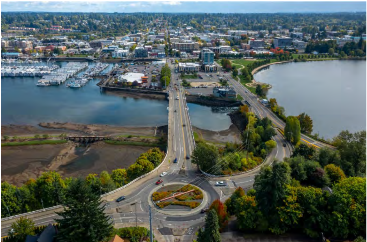
The lower roundabout that links the 4 th and 5 th Avenue Bridges to the westside.
