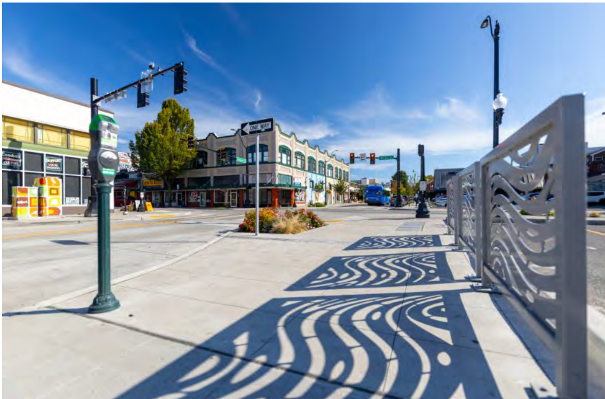
The rebuilt sidewalk on Franklin Street included some public art elements to make walking more inviting.
