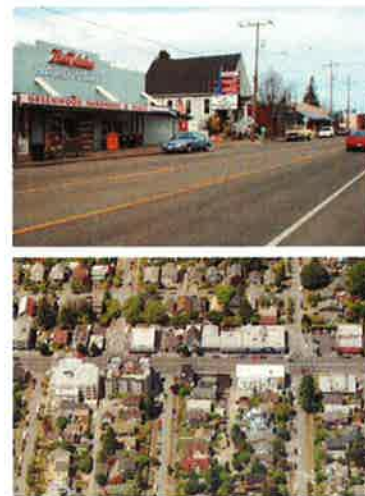
Figure 8. The Phinney neighborhood business district, anchored by an approximately 6,000-square-foot grocery and a 5,000-square-foot hardware store.
