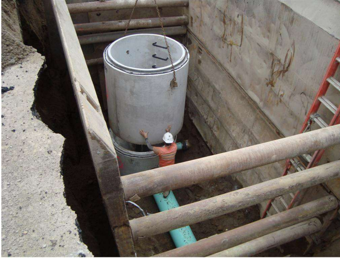
Installing a deep sewer maintenance hole on Henderson Boulevard as part of a planned capital improvement project.
