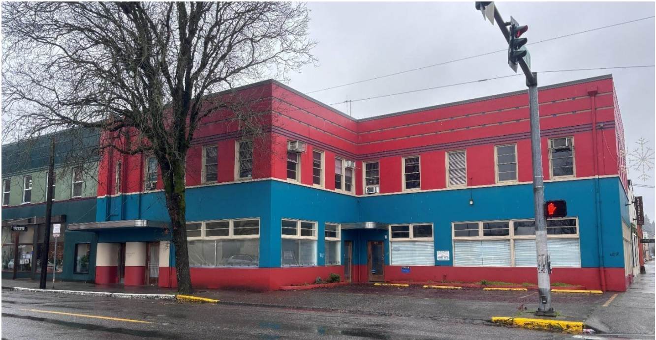
Figure 14. A Mostly Vacant Class C Office Building at 121 State Avenue NE
