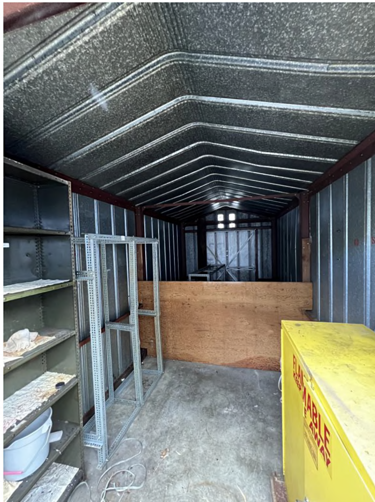
22 of 22 (WA_Thurston_NationalGuardArmoryOlympia_0012) Interior of Butler Shed at northwest corner of site.
