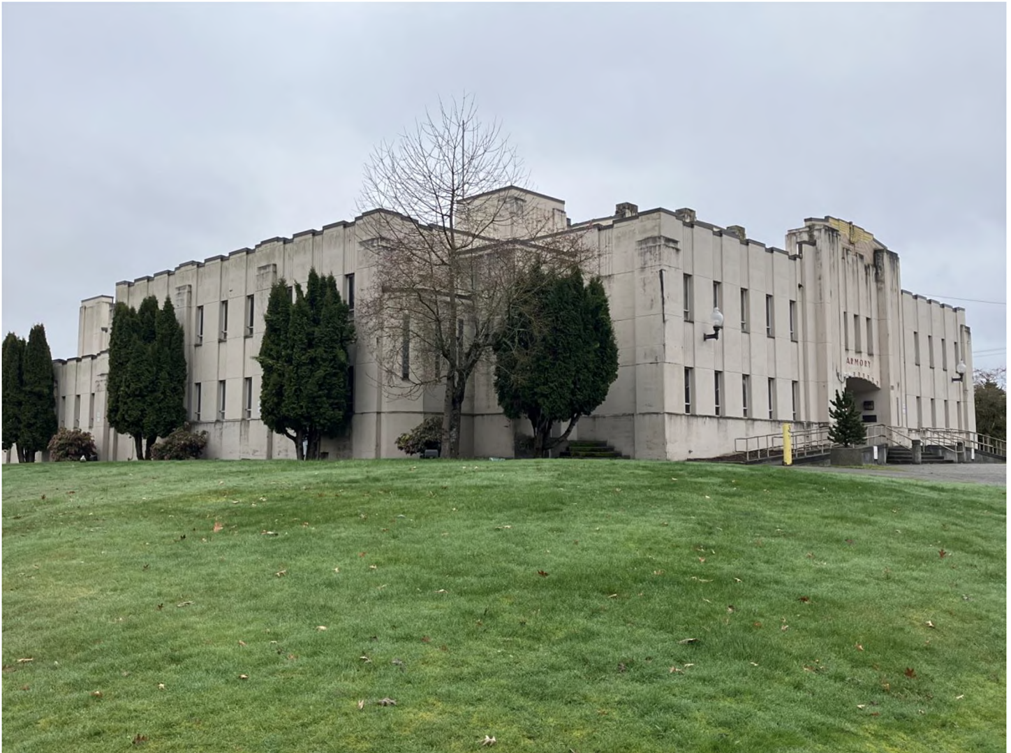
1 of 22 (WA_Thurston_NationalGuardArmoryOlympia_0001) View of the Olympia Armory looking northwest.
