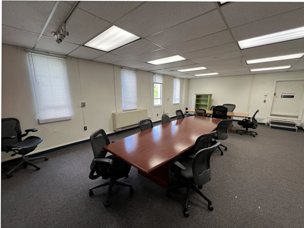
13 of 22 (WA_Thurston_NationalGuardArmoryOlympia_0008) Typical second floor office area.
