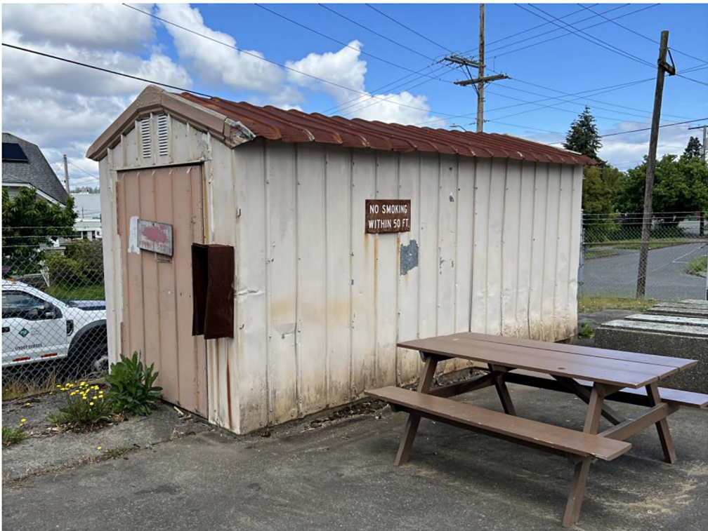
21 of 22 (WA_Thurston_NationalGuardArmoryOlympia_0011) Butler Shed at northwest corner of site.
