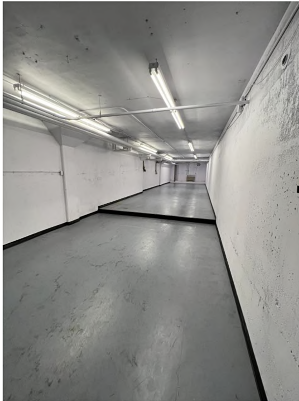
16 of 22 (WA_Thurston_NationalGuardArmoryOlympia_0010) Basement firing range - looking west.
