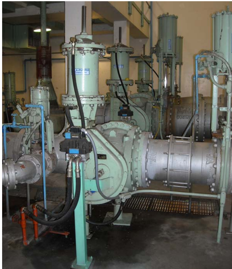
Figure 43. Example pump station having 40 cfs capacity
