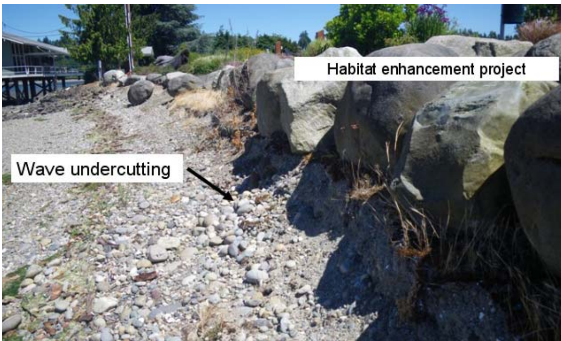
Figure 35. Shore protection and habitat enhancement features vulnerable to increasing level of wave damage
