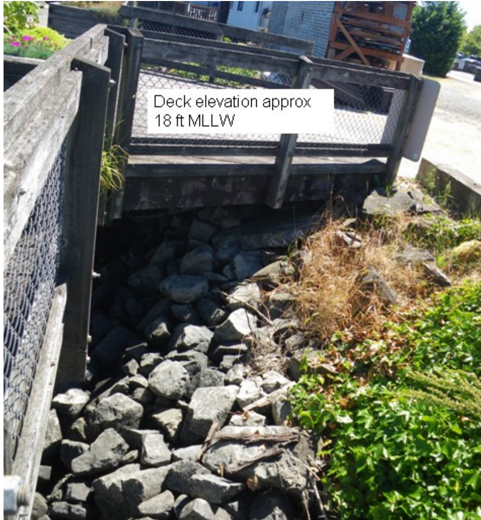
Figure 32. Fixed shore structure vulnerable to more frequent inundation
