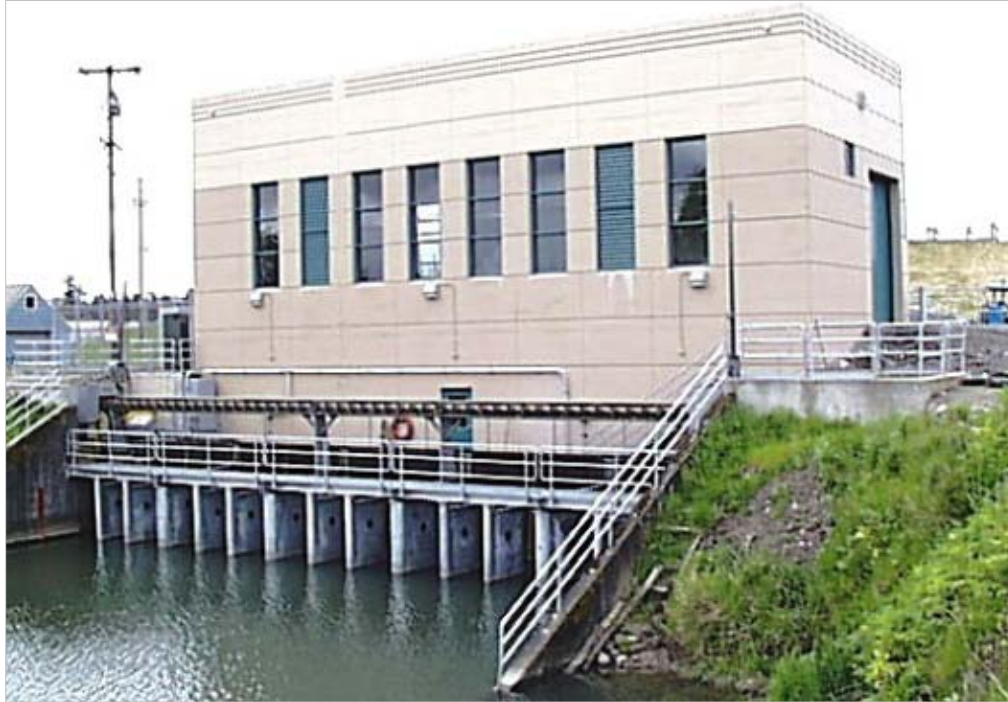
Figure 42. Example pump station having 500 cfs capacity
