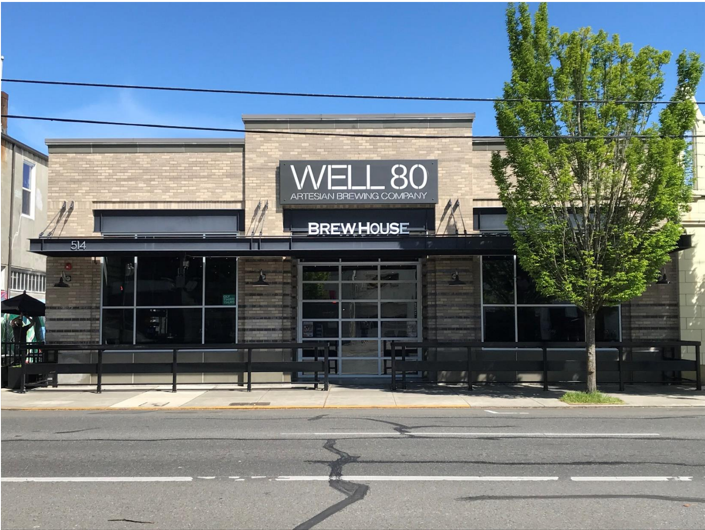
2019 Photo of Well 80 Building
