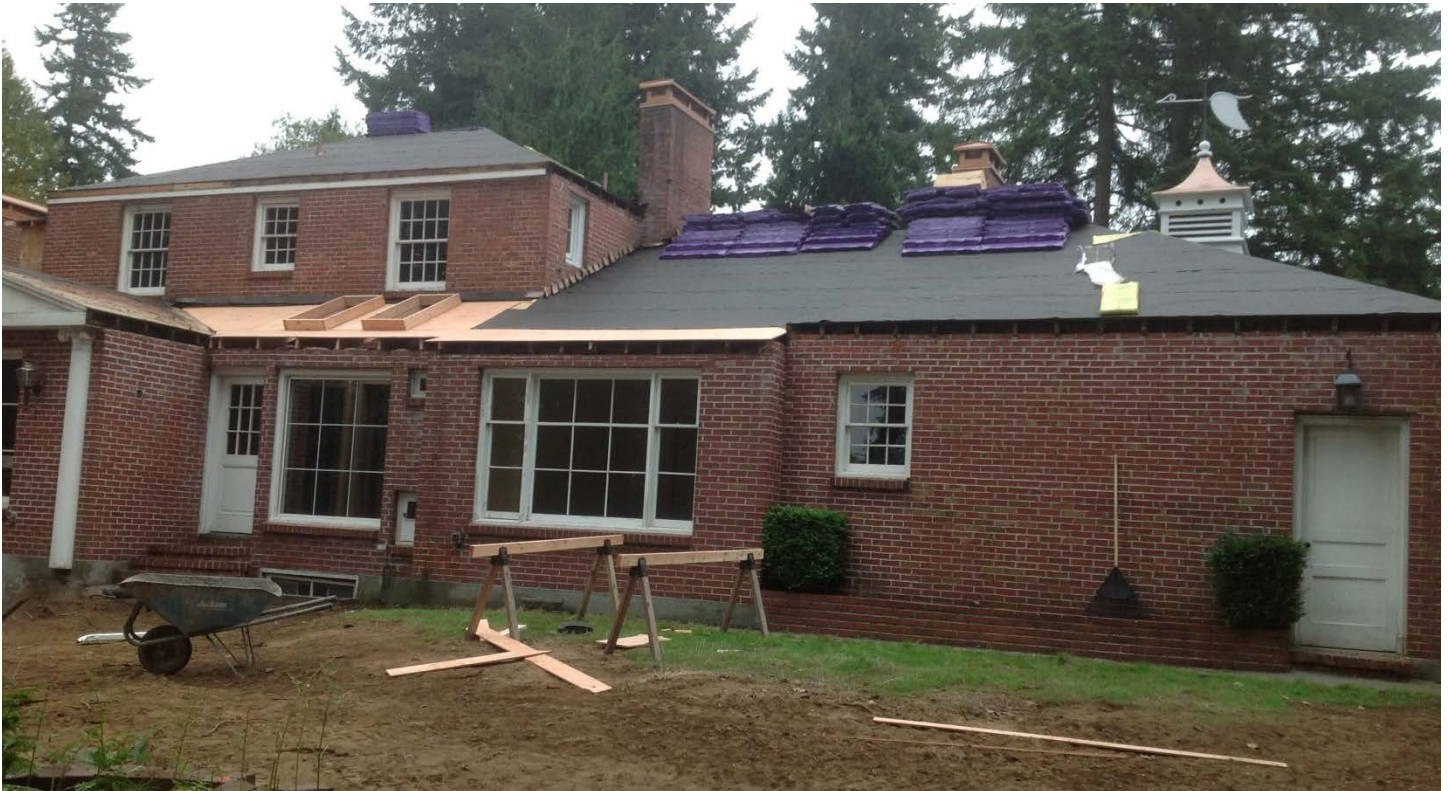
Complete reroof, gutter, and chimney rehabilitation.
