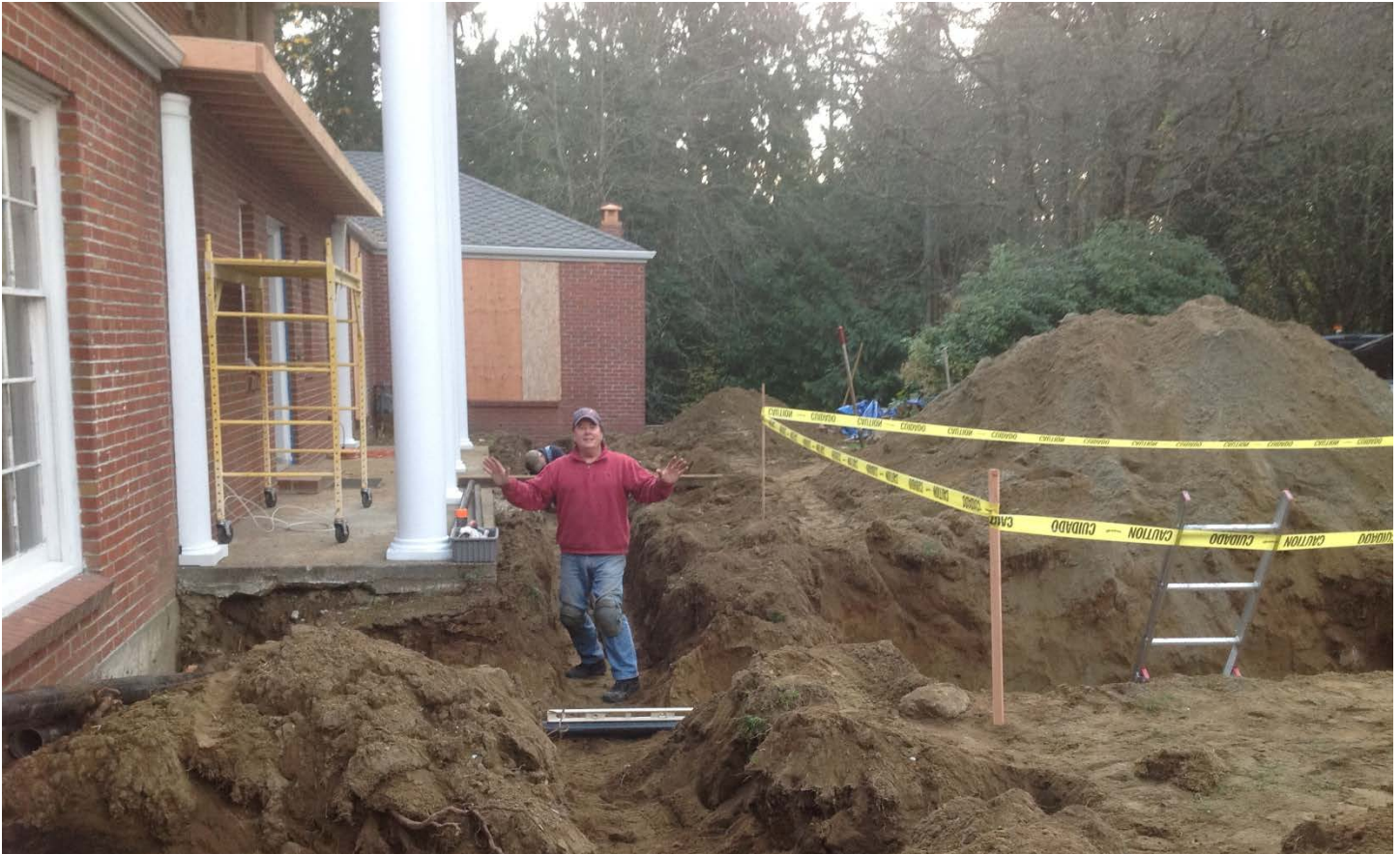
Sewer upgrades and rehabilitation work on the front porch and balcony.
