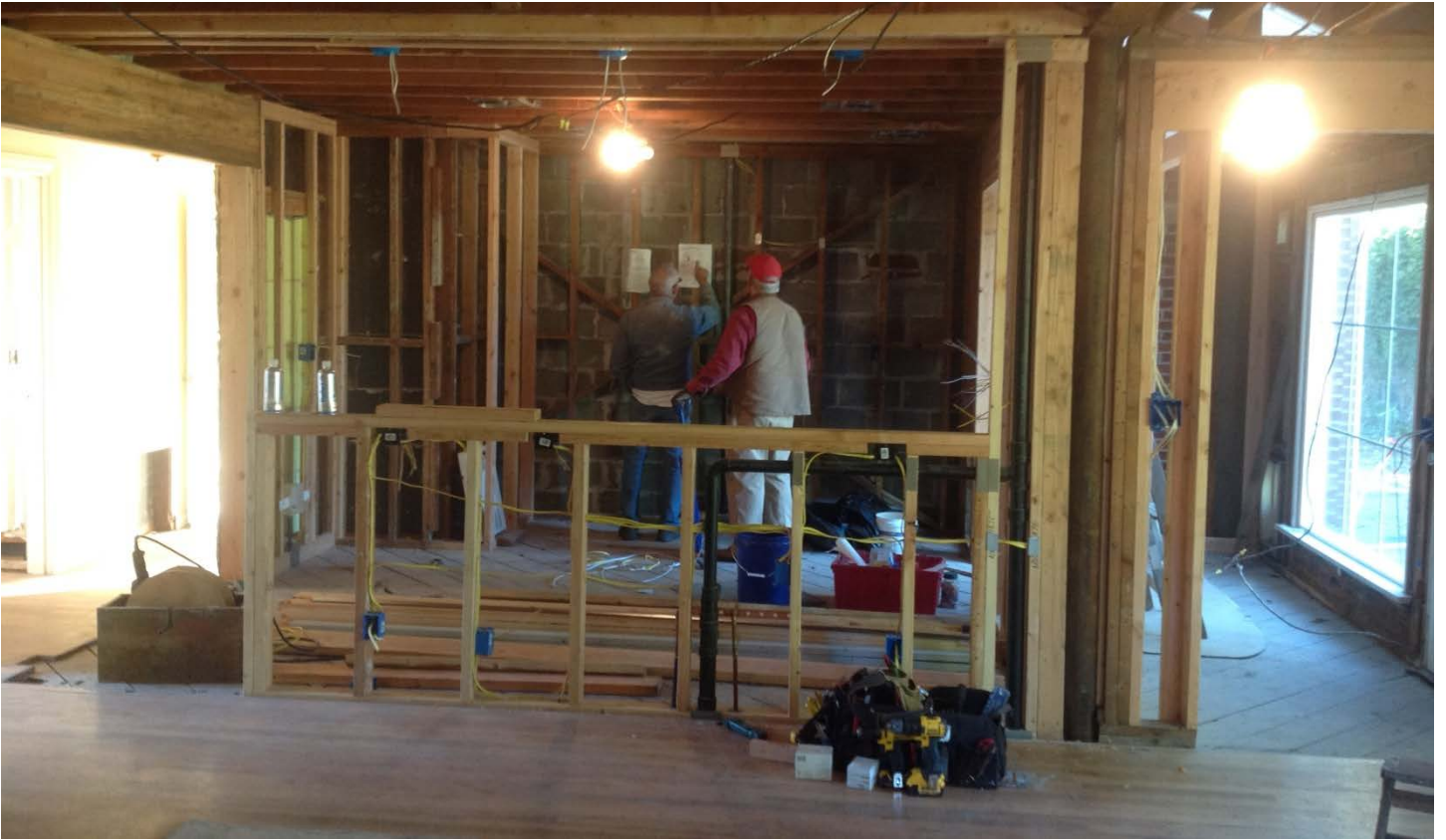
Framing the upgraded kitchen.
