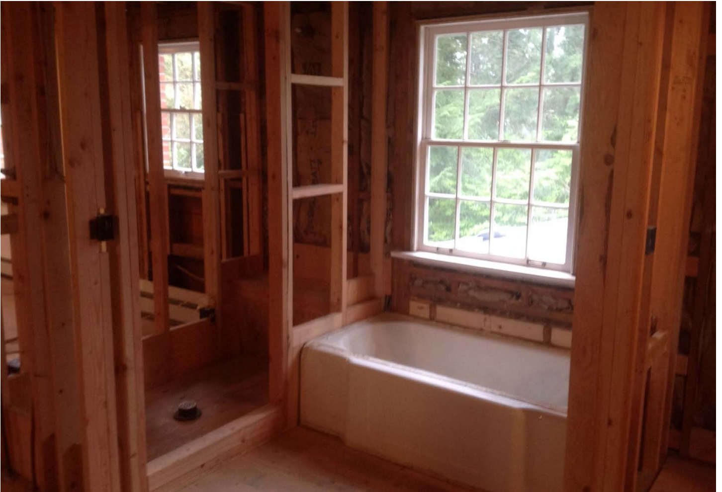
New master bathroom in the works.
