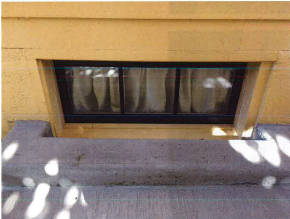
12 Exterior basement window with well 2016
