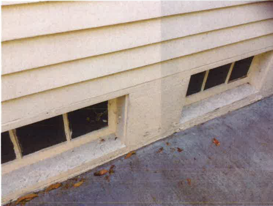
11 exterior basement windows 2015
