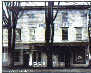
Pacific House, shortly before demolition, Roger Easton Collection
