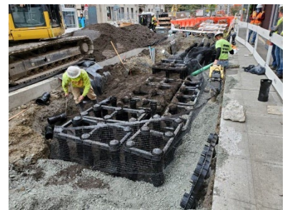
Figure 4-3. New technologies like soil cells allow for proper soil volumes for urban trees while still accommodating utilities, irrigation, and paving in tight conditions.
