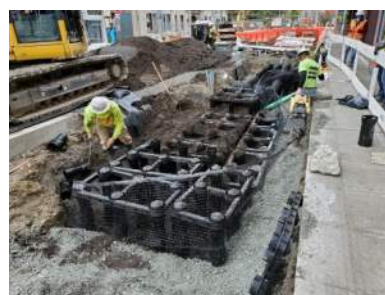
Figure 4-3. New technologies like soil cells allow for proper soil volumes for urban trees while still accommodating utilities, irrigation, and paving in tight conditions.
