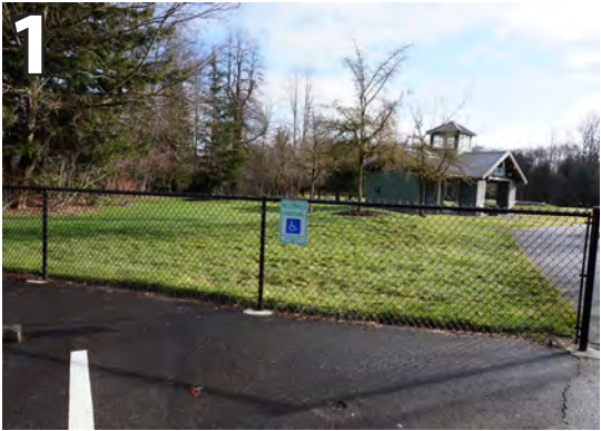
Provide van accessible sign and raise so bottom of sign is at 60"
