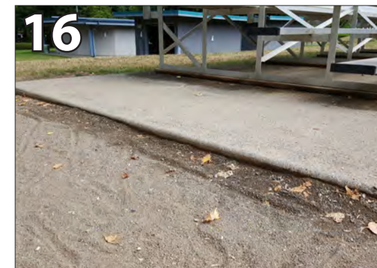
16 Spectator area not flush w/ crushed stone area.
