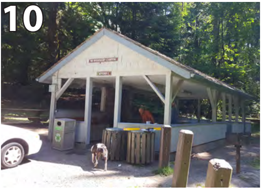
No ADA parking. Shelter threshold exceeds 1/2". Provide (1) ADA parking space. Install ADA pathway from ADA parking space to shelter.
