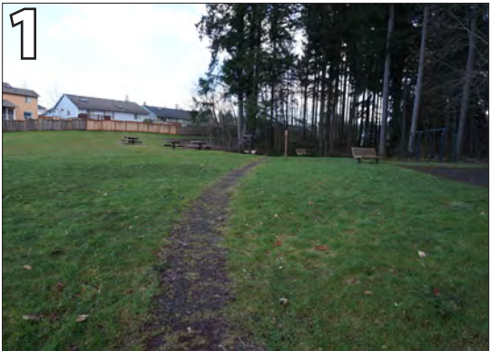
1 Existing pathway is worn and narrows to 24" for large portions of its length. Replace with ADA compliant pathway.
