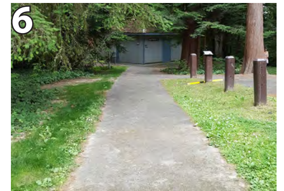
Running slope is greater than 1:20 and cross slope exceeds 1:48. Asphalt has surface bumps greater than 1/2". Regrade and resurface.
