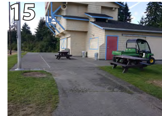
Slope exceeds 1:20 and is considered a ramp. Install railings on either side of ramp.
