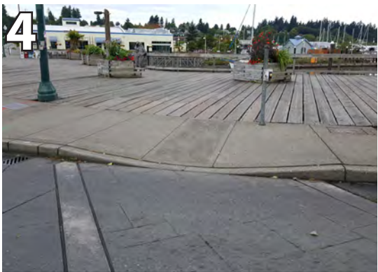
Curb ramp not ADA compliant. Regrade curb ramp.
