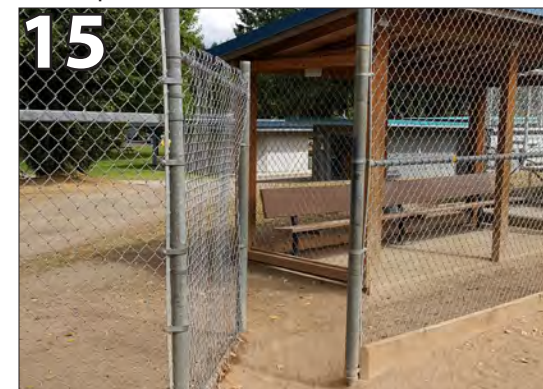
15 Fence opening too narrow. Widen to 36".
