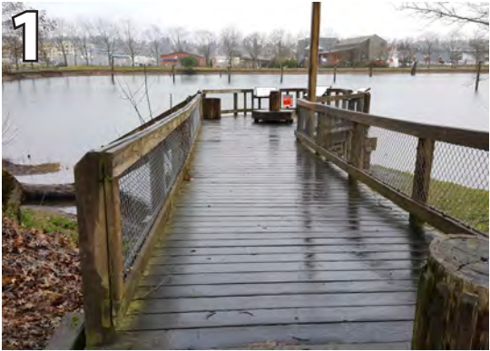
Decking is very slippery do to build up of moss. Implement a more frequent maintenance program or coat with anti-slip product.
