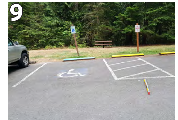
Running slope and cross slope of access aisle are not compliant. Install ADA compliant parking sign. (Sign has been removed since this picture was taken.)
