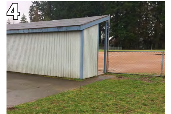
Pathway to dugout opening is too narrow. Widen to 60".
