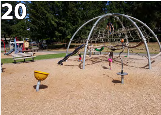
20 EWF is very worn down in both play areas. Especially around the play equipment making the spaces non-ADA compliant.
