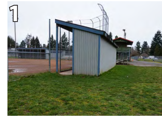
No ADA access into dugout on Field #2 from outside the field. Install ADA complaint pathway from existing asphalt to dugout opening.
