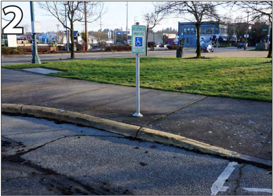
Provide van accessible sign at proper height.
