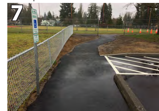
Raise sign so bottom of sign is at 60".
