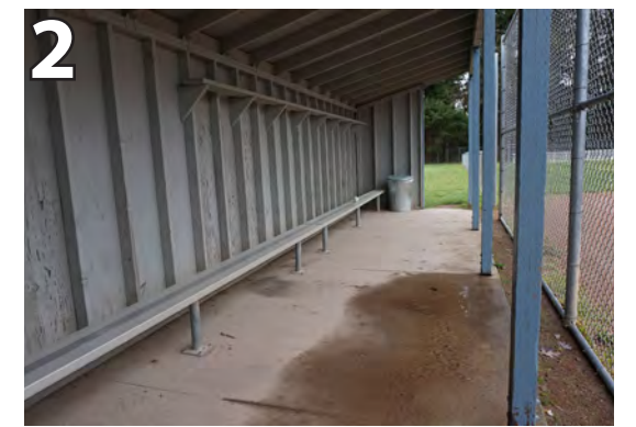
No wheelchair space in player seating for all 4 dugouts. Create opening that is centralized and at least 48" wide.
