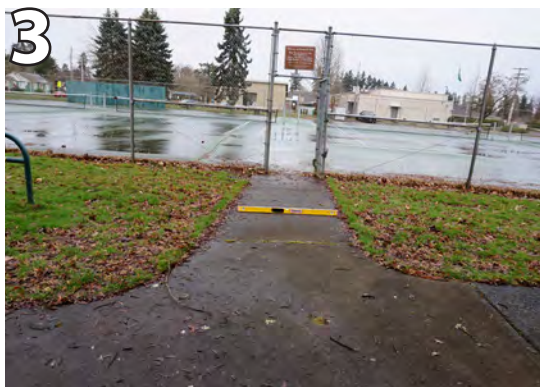
3 Pathway leading to tennis courts has a running slop of 6.6% and cross slope of 6.1%. Regrade pathway to be ADA compliant.
