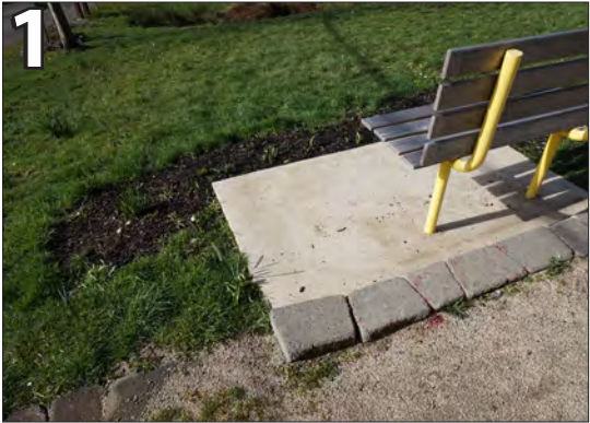
Expand concrete slab to allow room for a wheelchair and improve access from crushed stone pathway.
