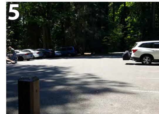
Inadequate ADA parking. Provide (1) ADA accessible parking space with proper signage
