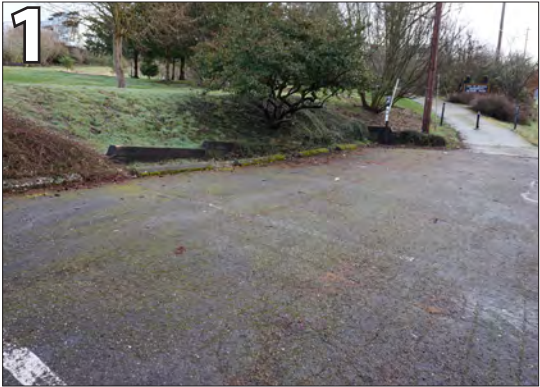
No ADA parking. Provide (1) ADA compliant parking space that has proper grade, markings and signage.
