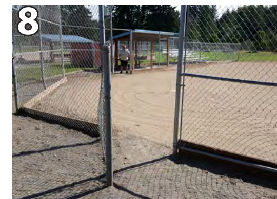
8 Widen fence openings to 36".
