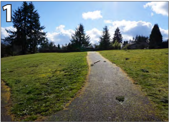
Running slope exceeds 5% and cross slope exceeds 2%. Regrade so pathway is ADA compliant.
