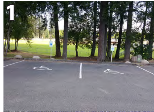
1 Inadequate access isles. Signage displayed too low. Provide proper access isles and proper signage.
