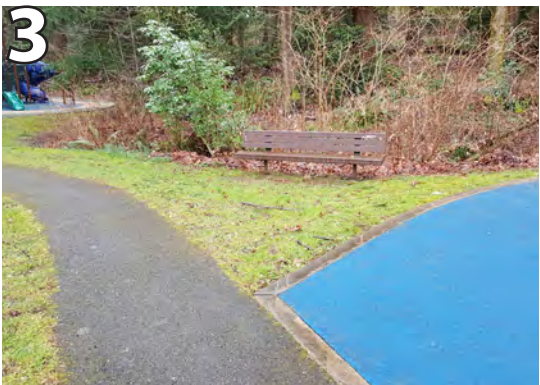
Bench is not accessible. Add accessible route to bench and provide 36" x 48" level pad on one end of the bench.
