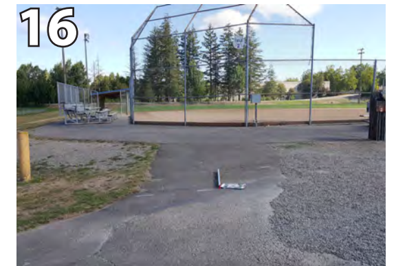
Running slopes and cross slopes are not compliant. Re-grade and resurface,
