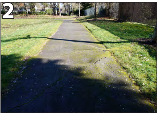
Tree roots are pushing up asphalt trail in excess of 2"+ in several places along this length of path.
