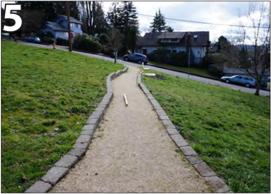
Regrade so that cross slopes are 1:48 or less.
