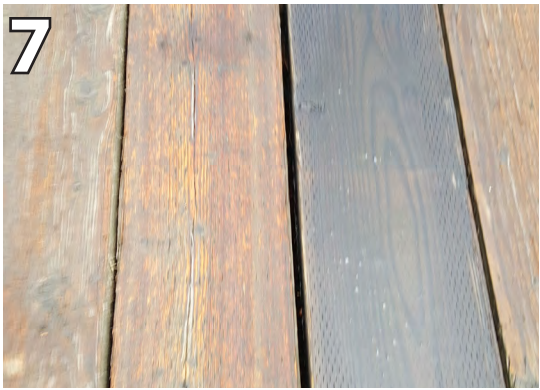
Openings between boardwalk planks were measured up to 2" wide.
