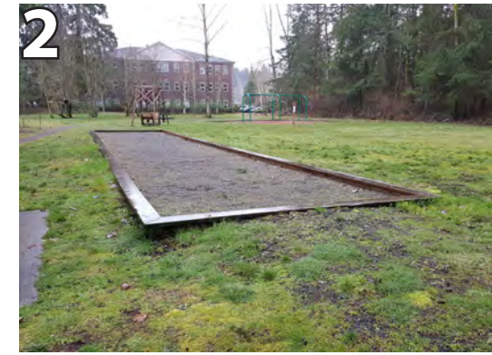
2 Bocce ball court not accessible. Add accessible pathway to court and provide accessible method of entry to allow for access into court.
