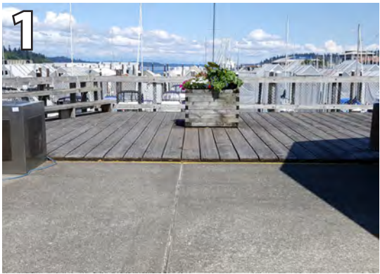
Entrance onto boardwalk to high. Regrade sidewalk to be flush.
