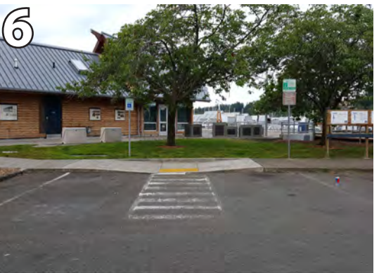
Inadequate ADA parking. Provide (3) ADA accessible parking spaces. (1) must be van accessible and have proper curb cuts & signage.
