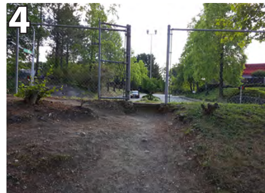
4 Park entrance not ADA accessible. Provide ADA accessible pathway that is flush with the sidewalk and connects to path below.
