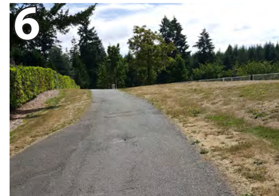
Exceeds 1:20 running slope and 1:48 cross slope. Regrade and repave.
