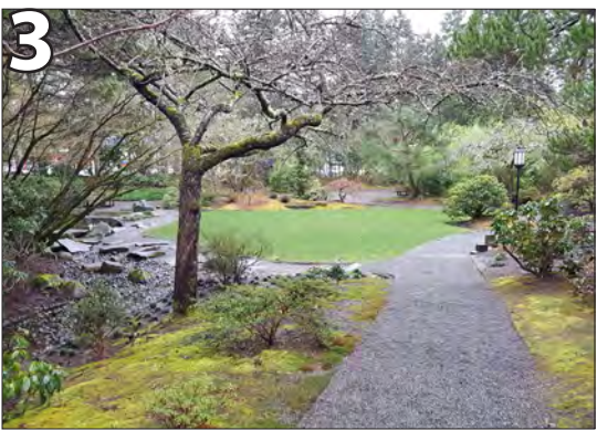
Cross slope near trail intersection is 3.5%. Regrade so cross slope is less than 2.08%.
