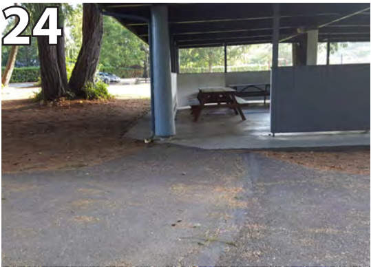
24 Regrade entrance of picnic shelter so that the asphalt and concrete pad are at the same grade.
