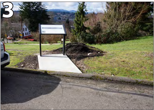
Provide curb ramp to allow for access to signage.
