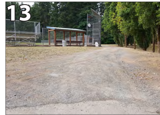
13 Non-compliant slope and surface. Re-grade to a slope no greater than 1:20 and replace surface with asphalt.
