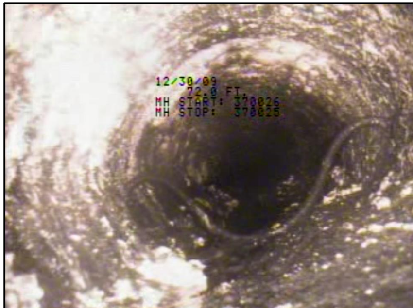
Figure 8.1 Example of a lined gravity sewer pipe
