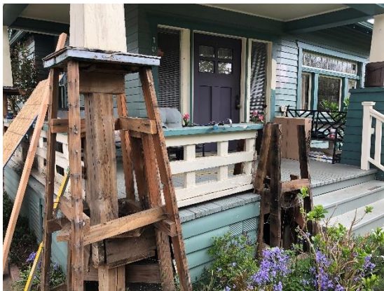
Front piers, siding removed
