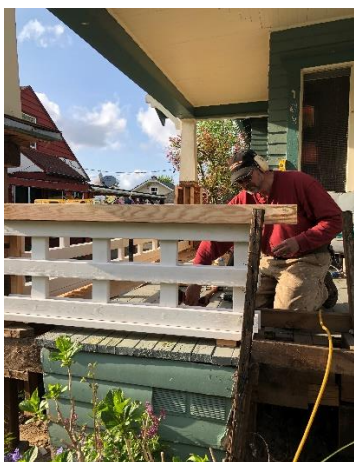
Building and installation of new porch railing
