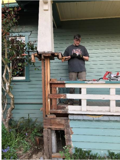
Removal of rotten clapboard siding on piers
