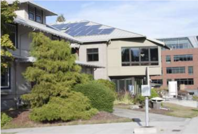
Solar panels on a commercial building in downtown Olympia.
