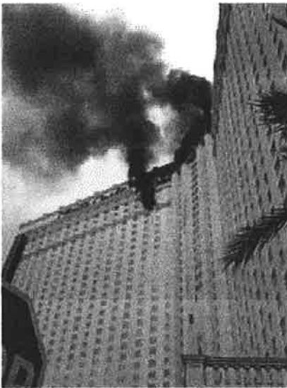
(6) The Monte Carlo Hotel fire involved EIFS installed on the exterior of the building. ( Photo by Dave Connell. )
