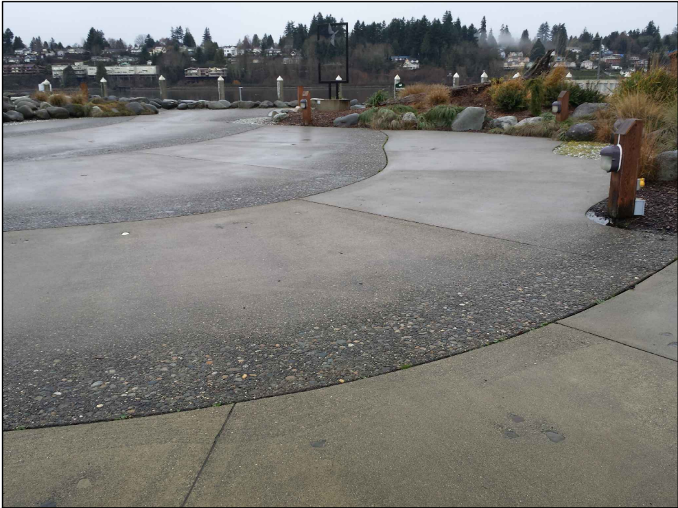
Beach-look exposed aggregate concrete
