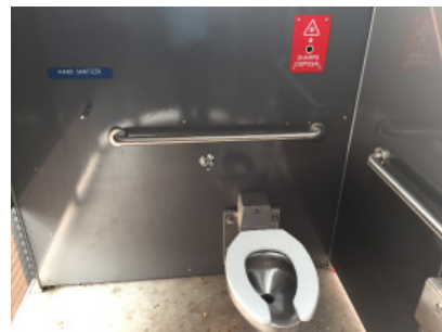
Through wall sharps disposal at the new Portland Loo
