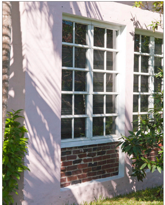
The small holes along the top and bottom of the window allow quick installation of fabric storm panels and are visually inobtrusive.
