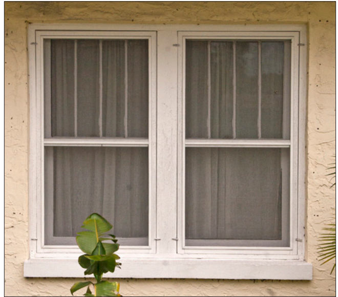
The horizontal rail of the window screens align with the meeting rail of the window. The clip-in attachment allows for a visually minimal frame.
