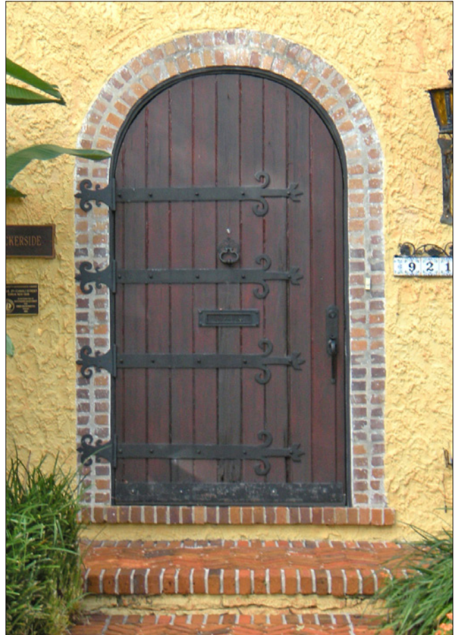
Front doors should complement the style of a building. This wood plank door with heavy iron straps is appropriate for the Mediterranean Revival residence.
