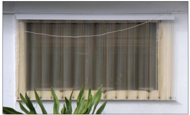
The corrugated Plexiglas in this example has yellowed and obscures the window. It is not appropriate at a historic building.
