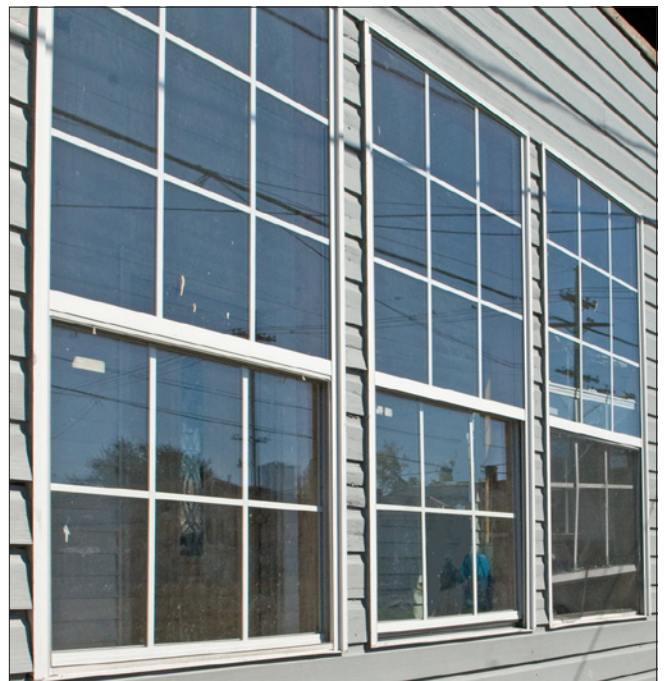
The 9-over-6 vinyl replacement windows have applied muntins, are mounted flush against the outside wall and lack the depth of traditional windows. They do not have trim or casings. They are not appropriate for historic buildings.
