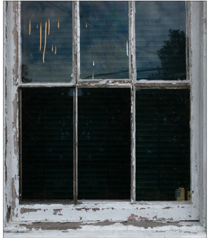
Often, the deterioration of wood windows first occurs at the sill. Peeling paint can allow moisture to enter wood and cause rot. Regular repainting is recommended to provide a protective layer against moisture.
