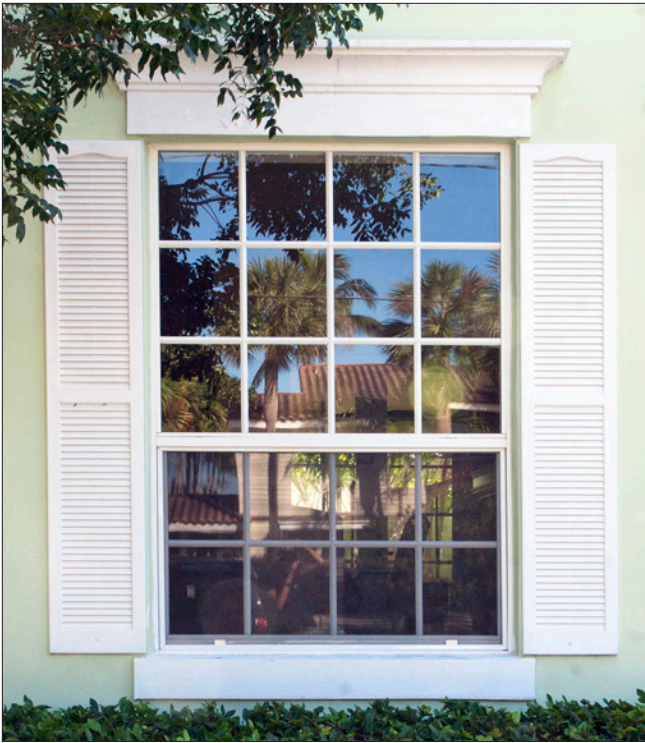
Shutters should be operable and proportioned to fit the window. The shutters in this example are fastened to the side of the building and too narrow for the window opening.
