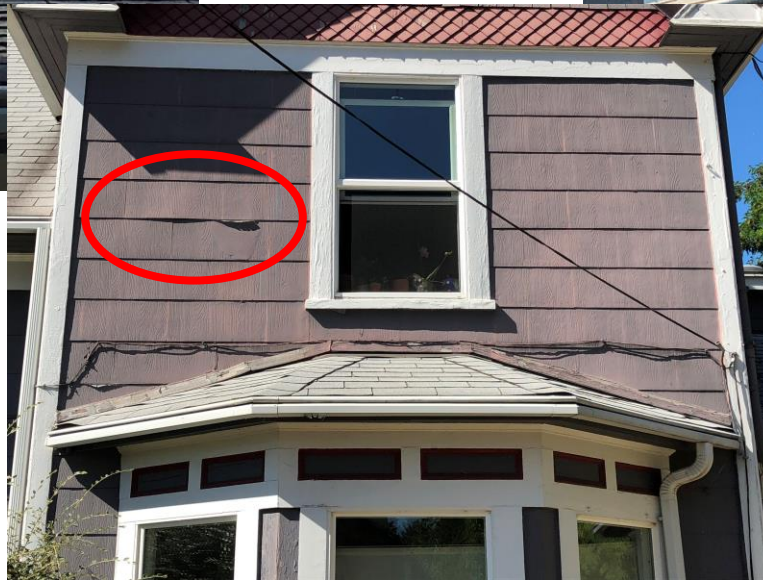
Examples of damaged siding to be replaced
