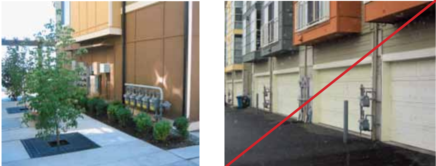
Good and bad utility meter configurations. The example on the left is consolidated and somewhat screened by landscaping elements, whereas the right example is exposed and degrade the character of this project.
