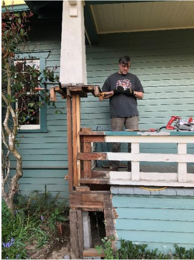
Removal of rotten clapboard siding on piers
