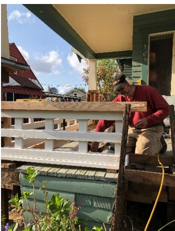
Building and installation of new porch railing
