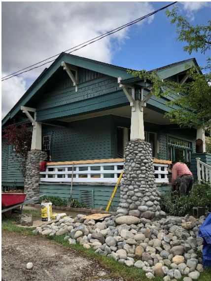
River rock piers built by hand
