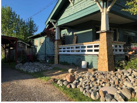
New porch railing installed, piers stabilized and wrapped in OSB
