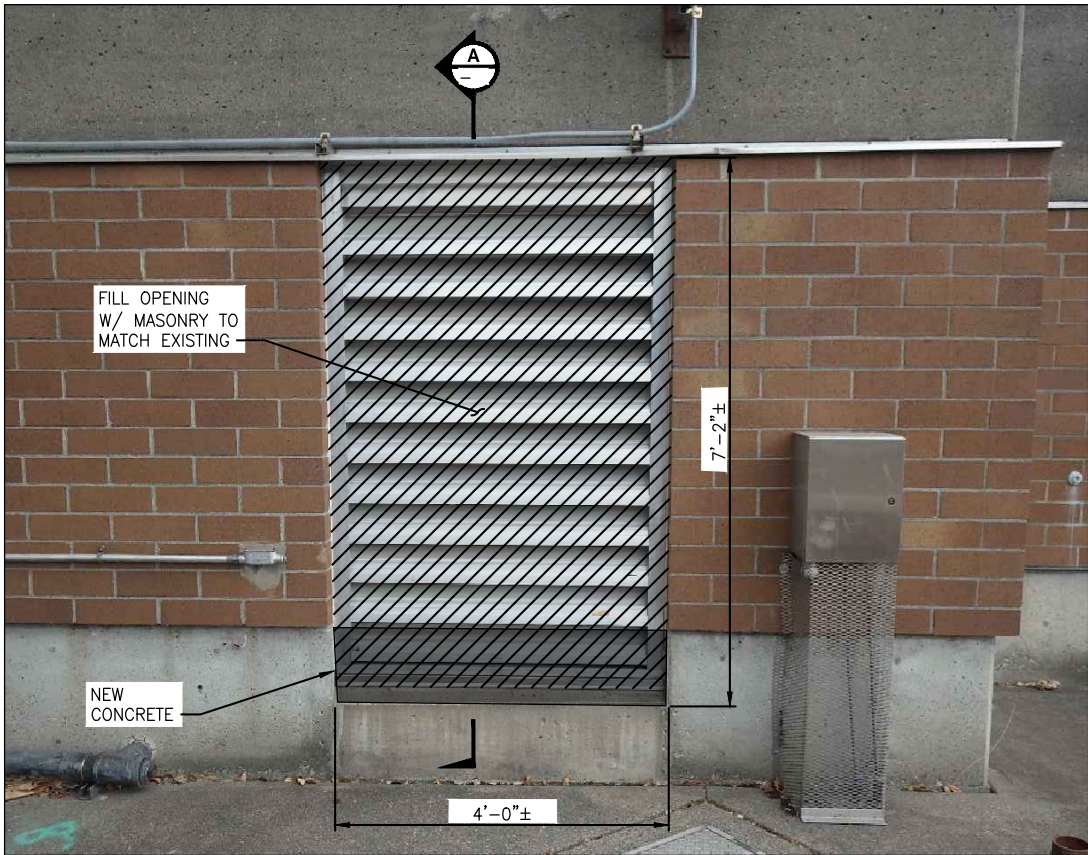
SOUTH LOUVER DETAIL NO SCALE
