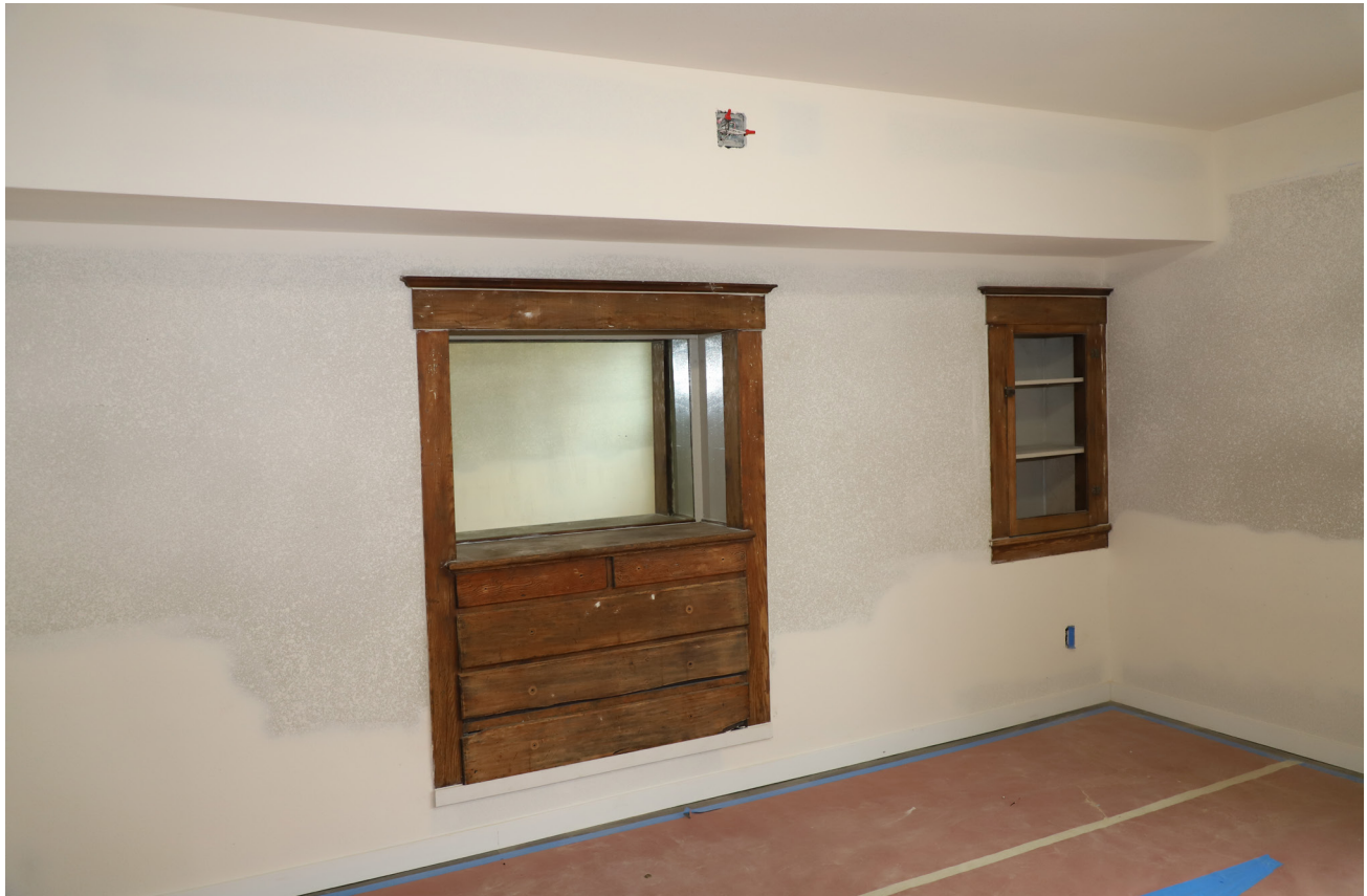
Photo 65. After, 2021, unit 301 retained built-in cabinets, sanded and prepped for painting.
