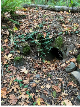
Photo 13: Seasonal Stream 1 culvert #1, Central Mainline Trail, October 2025.
