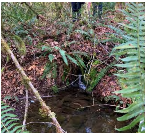
Figure 6. Downstream of central culvert with plunge pool.
