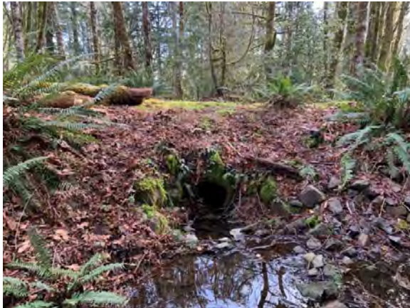
Figure 4. Upslope side of culvert crossing at central trail.
