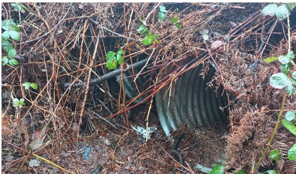
Photo 5: North end of existing culvert under access road, February 2025.
