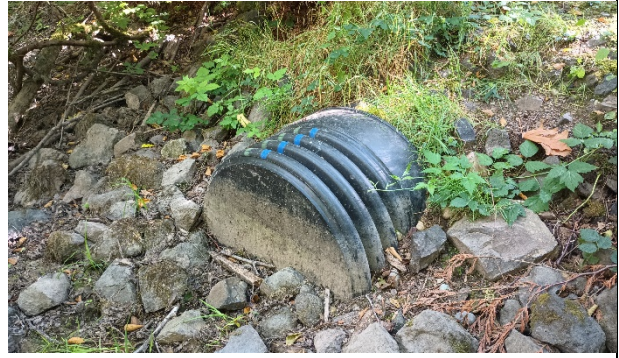
Photo 14: Seasonal Stream 1 culvert #2 (capped), Central Mainline Trail, July 2025.
