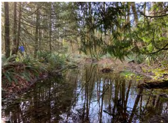
Figure 5. Ponded area on upslope side of culvert crossing.
