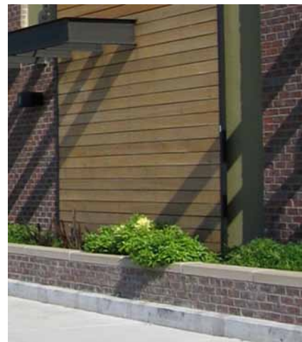
Building detailing & raised planter
