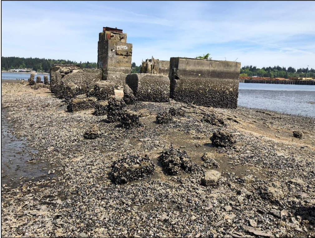
Photograph 6. Large concrete structures, debris and piling to be removed, located immediately waterward of property shoreline.
