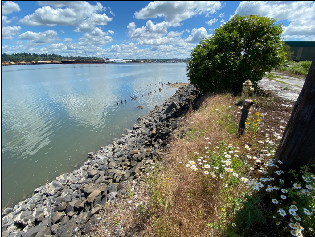
Figure 7. View southeast along waterline showing gravel slope with old pilings in adjacent property.
