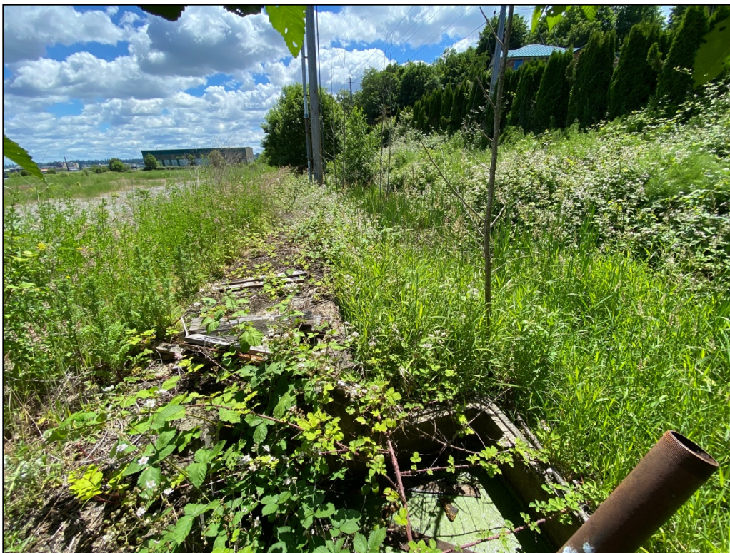
Figure 6. View south along the rail platform on the east edge.
