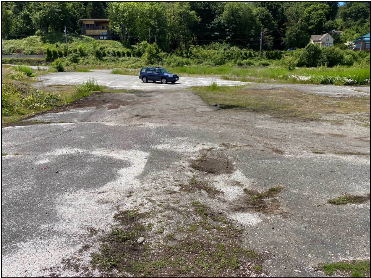
Figure 4. View west, over concrete pad.
