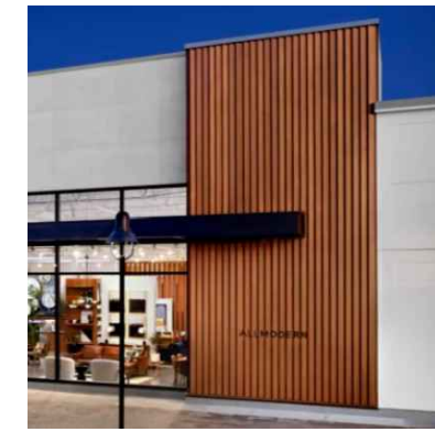
MAIN ENTRY ELEMENT: WOOD-LOOK VERTICAL PANELS FULL-HEIGHT TO ACCENTUATE THE ENTRY & BRING THE EYE UPWARD
