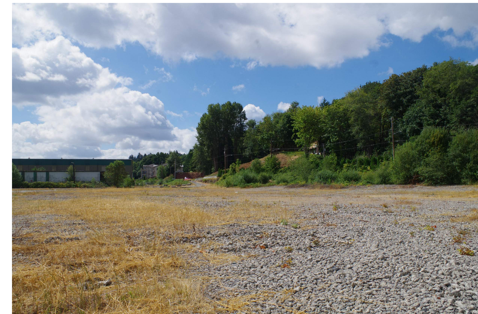
LOOKING SOUTHWEST TOWARDS EXISTING RESIDENCE
