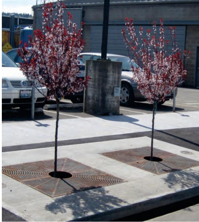
Figure 5 - Filterra® Bioretention System installed adjacent to sidewalk
