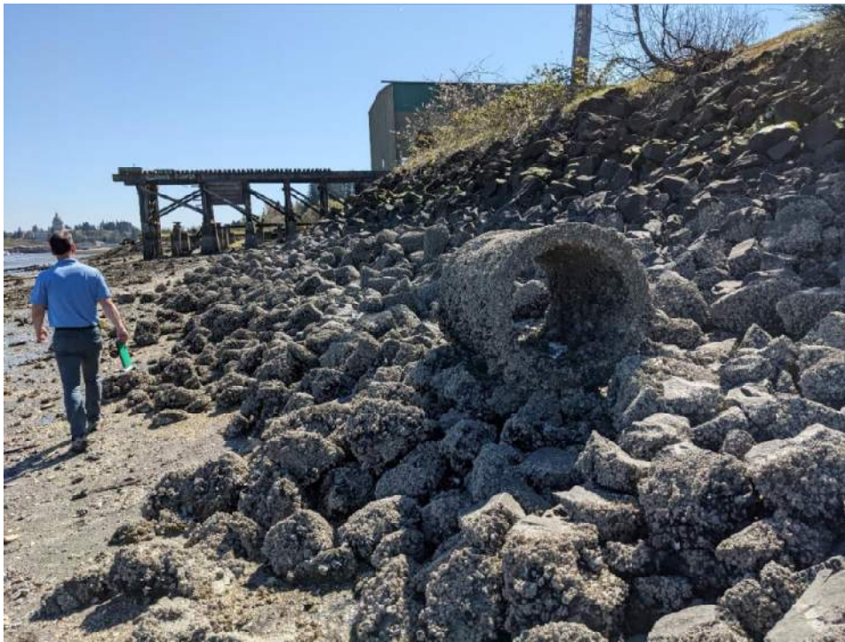
FIGURE 2-5: STEEP, IMPACTED SHORELINE
