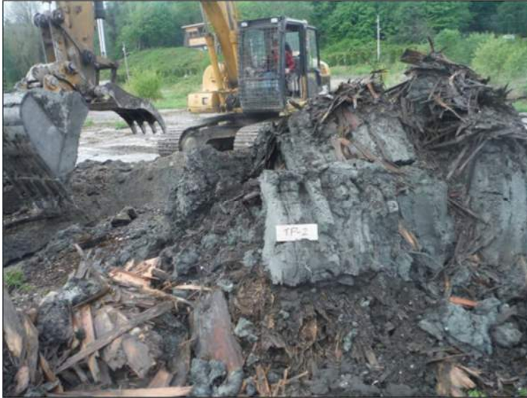
FIGURE 4-5: WOOD WASTE OBSTRUCTIONS IN TEST PIT 2 (LANDAU 2020)
