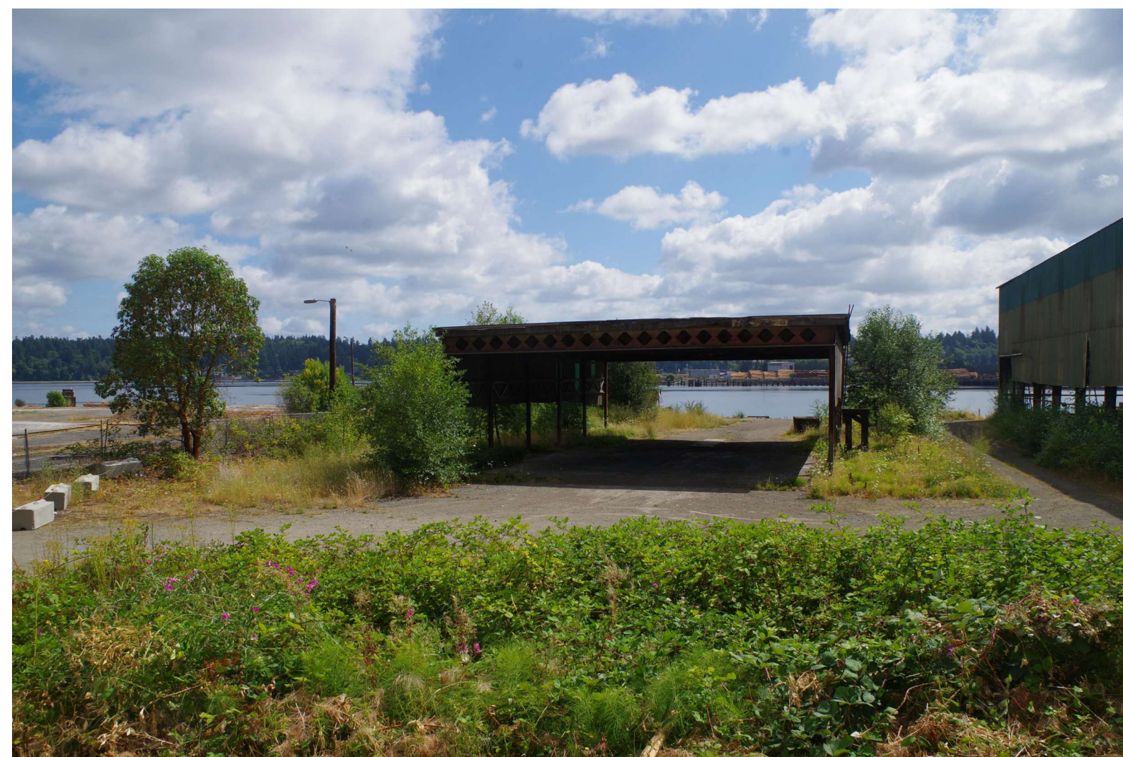
EXISTING ADJACENT ABANDONED STRUCTURE LOCATED SOUTH OF SITE
