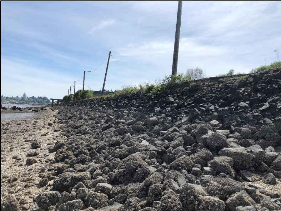
Photograph 4. Typical steeply sloping shoreline armoring along shoreline slope.
